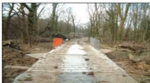
Ground protection image 6: Custom designed sectional tracks can be joined to support very heavy traffic use through sensitive areas.
