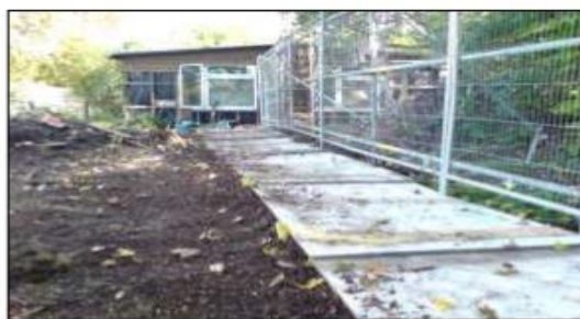
Ground protection image 1: Heavy-duty plywood set onto a compressible woodchip layer and pinned into position is suitable to spread the loading from pedestrian access.
