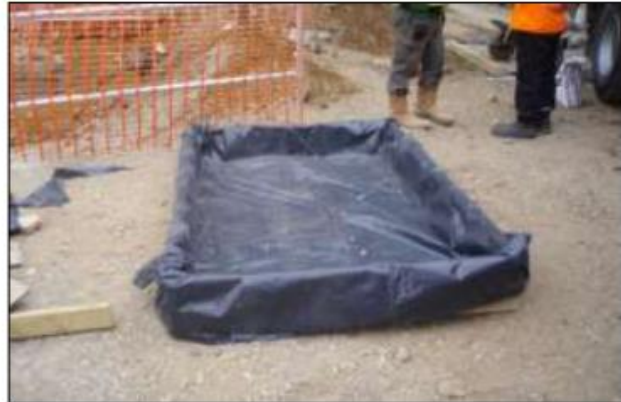
Pollution image 2: Soil bunding or a supporting framework covered in heavy-duty plastic sheeting is essential where there is a risk of spillages contaminating RPAs. This specifically applies to cement mixing areas and vehicle washing facilities.
