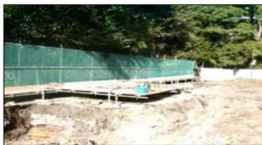
Ground protection image 4: A scaffold framework attached to the main scaffold fencing can be used to support either scaffold planks or plywood to create an elevated platform with a gap beneath.
