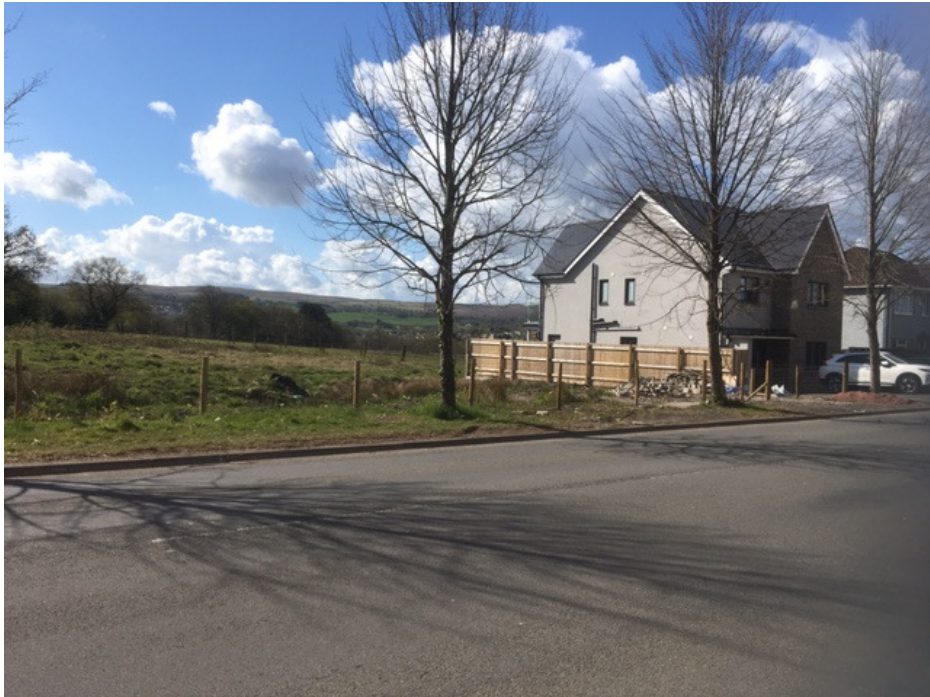
View of site and newly built detached dwelling.
