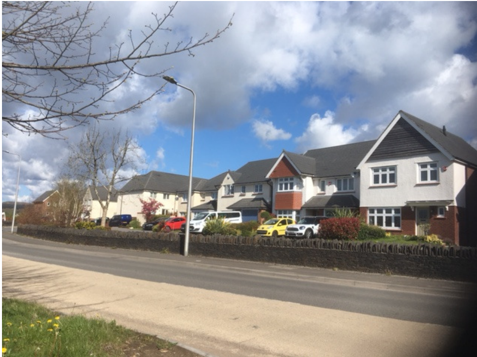
Photograph from road of Manor View
