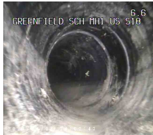
S18X_3237d3fb-c1ef-4f8b-88a7-18ec8fdef0ef_20210409_111551_334.jpg, 00:00:37, 6.70 m Line deviates left
