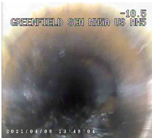
MH5X_acbd7248-6231-4b46-a672-8c097db1e455_20210409_1 121936_998.jpg, 00:02:34, 18.50 m Junction at 3 o'clock, diameter: 100mm
