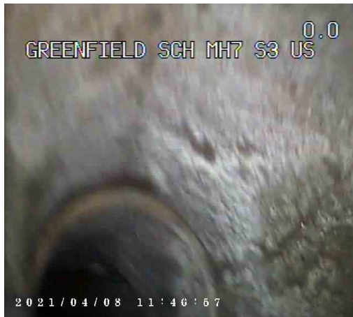
S3X_4ed7c991-3afb-4c49-a974-1f5c96bc161b_20210409_13 1207_659.jpg, 00:00:02, 0.20 m Line deviates left
