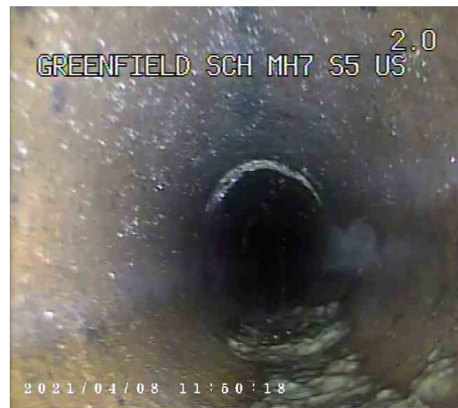
S5X_2d45addb-b2ca-400e-8ee0-89f7a52ac2d0_20210409_1 32450_858.jpg, 00:00:13, 2.00 m Settled deposits, coarse, 10% cross-sectional area loss, finish
