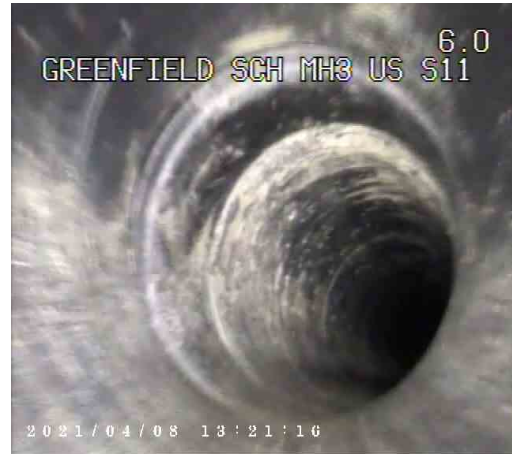
S11X_f74460b6-796b-4a6d-b9f2-52fe2d621ad6_20210409_1 15124_147.jpg, 00:00:32, 6.20 m Line deviates down
