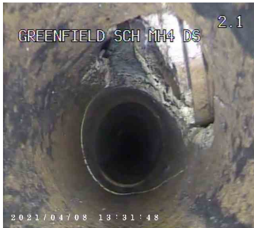
MH4X_7cdd99c8-6439-4cff-9660-40e9250bf3df_20210409_15415_579.jpg, 00:00:26, 2.20 m Connection other than junction at 2 o'clock, diameter: 100mm
