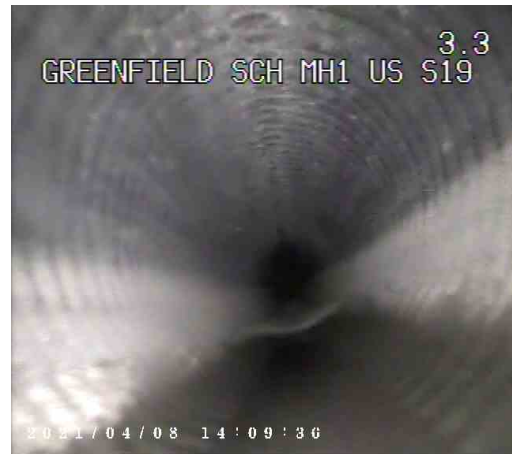
S19X_b1aa9b77-0b32-45b2-9359-86602c883dd9_20210409_112454_766.jpg, 00:00:15, 3.00 m Water level, 5% of the vertical dimension
