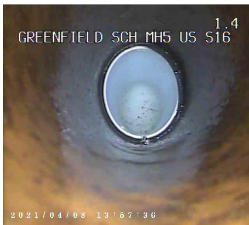
S16X_a93acb7b-ae4f-4e0e-a6d8-b49a16f0670c_20210409_1 52242_349.jpg, 00:00:14, 1.40 m Survey abandoned, End of line in building
