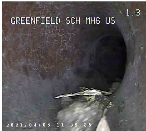
USX_7a828640-c1d6-4a7a-9674-9aaeb3a251d0_20210409_1 25454_260.jpg, 00:00:21, 1.50 m Line deviates right
