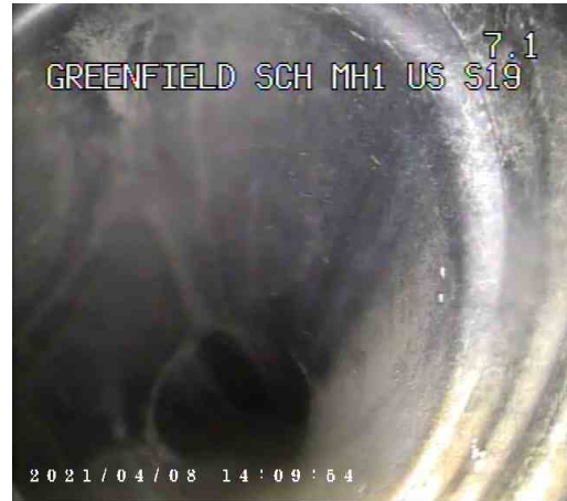
S19X_2e24307a-6ed1-441f-9c50-af9d07d74163_20210409_112930_845.jpg, 00:00:34, 7.50 m Line deviates down
