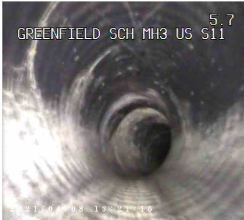
S11X_aa7399ee-ac2e-4dee-b6f6-cfd1c82ae481_20210409_1 15057_980.jpg, 00:00:31, 5.70 m Line deviates right
