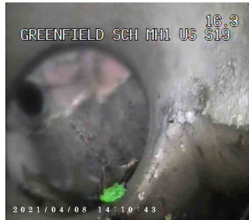
S19X_f1c9d01c-bf8b-4ac8-9bcf-4b6760874b71_20210409_11 3309_684.jpg, 00:01:22, 16.50 m Finish node type, gully, reference number: S19
