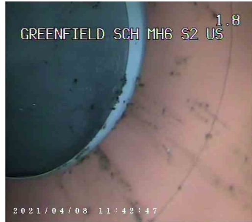
S2X_9e983243-242c-42f5-81ee-73fb63cb095e_20210409_13 0737_883.jpg, 00:00:24, 1.80 m Survey abandoned, End of line in building.
