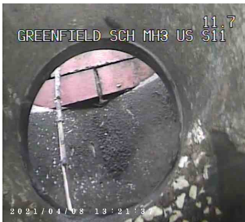
S11X_c5085f99-47e5-4918-93e6-d9c7a5a02d1b_20210409_1 115218_531.jpg, 00:00:54, 11.90 m Finish node type, gully, reference number: S11
