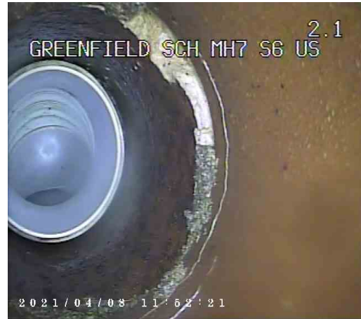
S6X_8a054d3d-90ad-4ea2-a2d0-509a61adccf9_20210409_1 32936_313.jpg, 00:00:19, 2.10 m Survey abandoned, End of line in building.
