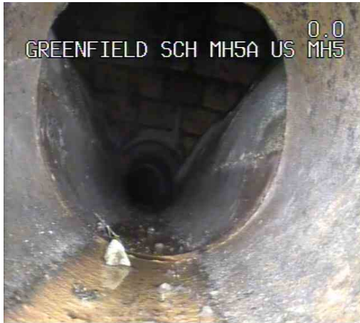
MH5X_857c9a79-cda8-431f-8440-64e2c46772c0_20210409_120159_034.jpg, 00:00:00, 0.00 m Start node type, manhole, reference number: MH5A
