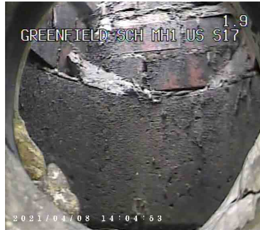
S17X_769ef3f8-d217-4f46-986e-247e8d287586_20210409_111403_878.jpg, 00:00:34, 2.00 m Finish node type, gully, reference number: S17
