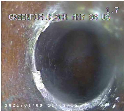
S6X_84fb33d9-67fd-4f7f-b726-649c8c28c2d8_20210409_133 009_859.jpg, 00:00:18, 1.80 m Line deviates up
