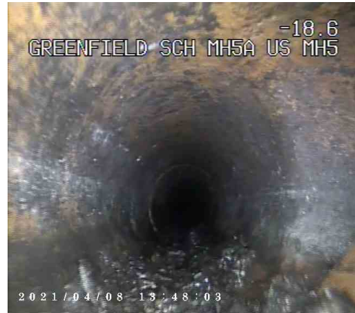
MH5X_98f16bd1-912f-44fa-8bb7-95dae7ce9453_20210409_1 21930_336.jpg, 00:02:34, 18.50 m Junction at 3 o'clock, diameter: 100mm
