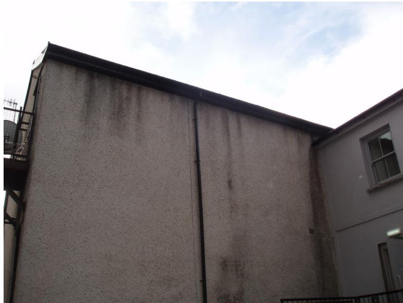
North facing elevation, new soffit, tightly sealed
