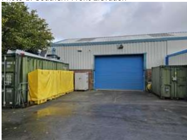
Photo 1: Southern Front Elevation
