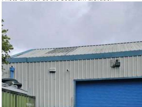
Photo 2: Roof at the Southern Elevation
