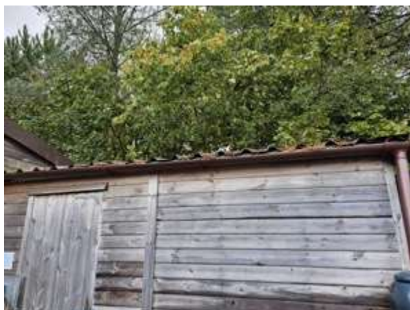
Photo 9: Roof at the North-Western Elevation
