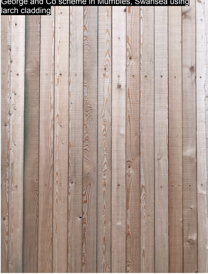
larch cladding with 10mm gap left to weather
