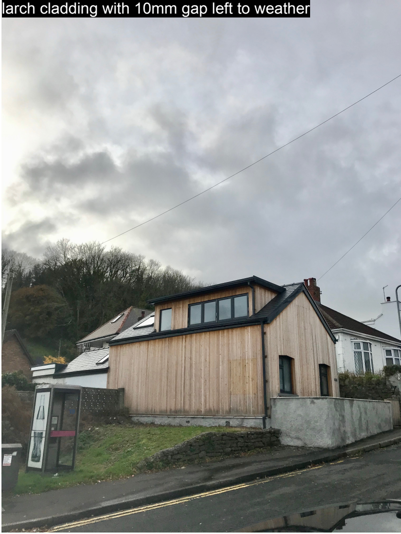
larch cladding with 10mm gap left to weather
