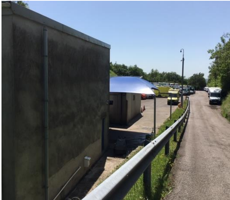
5. View south in to the Lower Yard (Valet buildings visible to LHS)
