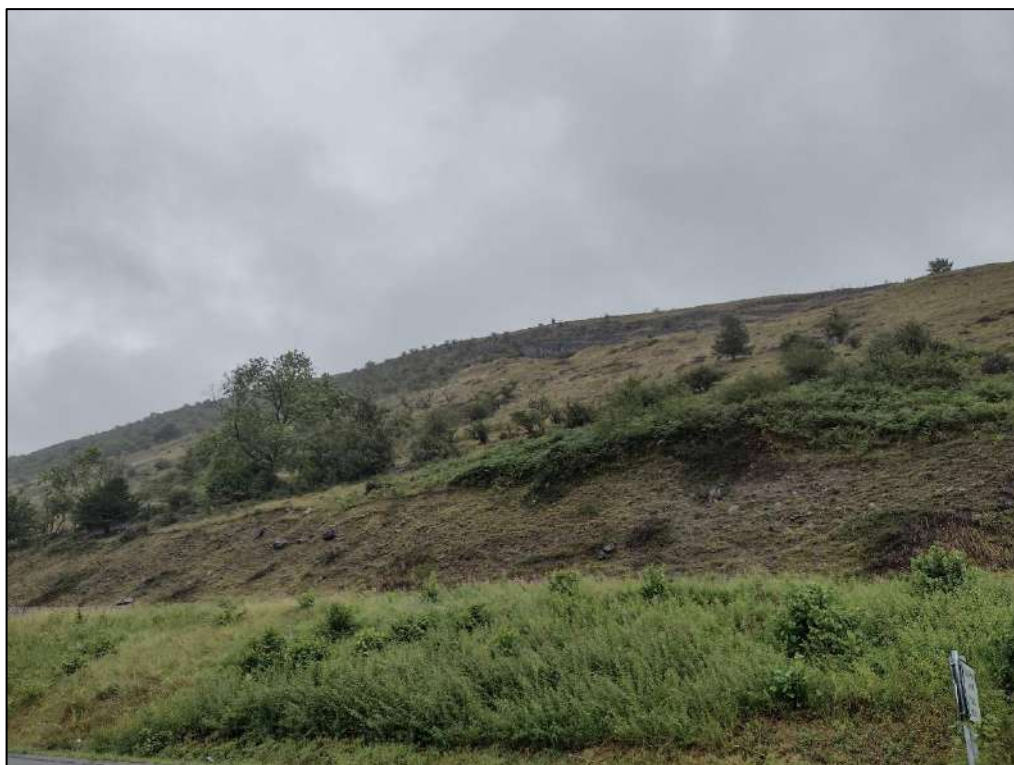
Photo 10. Cefn Cil-Sanws, facing north-east towards the Site
