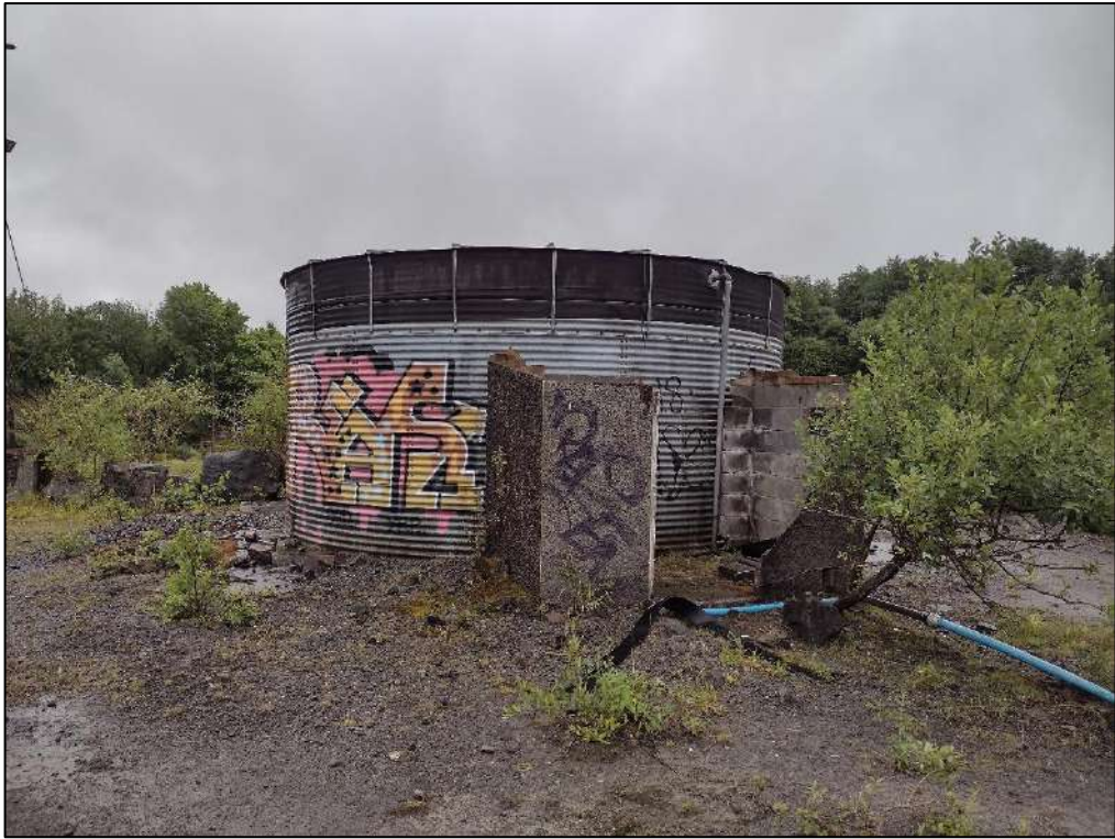
Photo 2. Storage tank, north facing elevation
