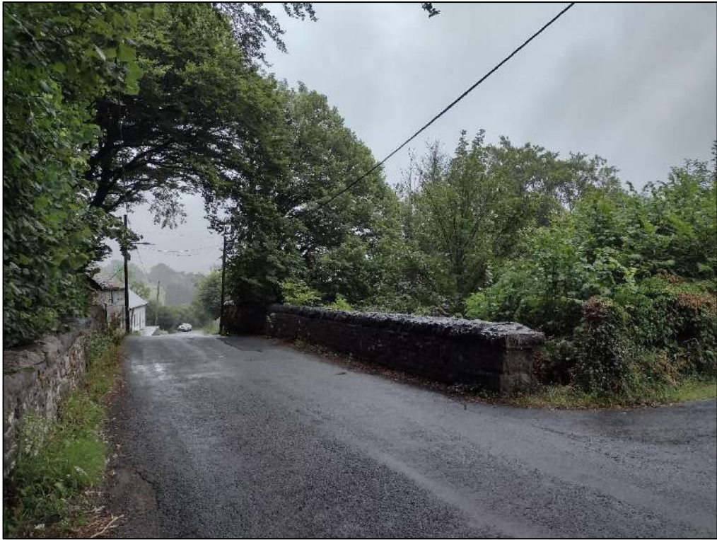
Photo 15. Road bridge near former Pontsarn Station (Fig. 3, LB2), looking south-west
