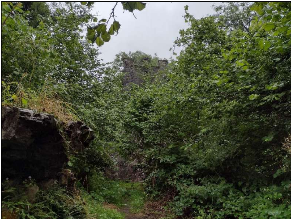
Photo 18. Tower of old church (St. Gwendoline) (Fig. 3, LB5) within area of dense woodland, looking south-east
