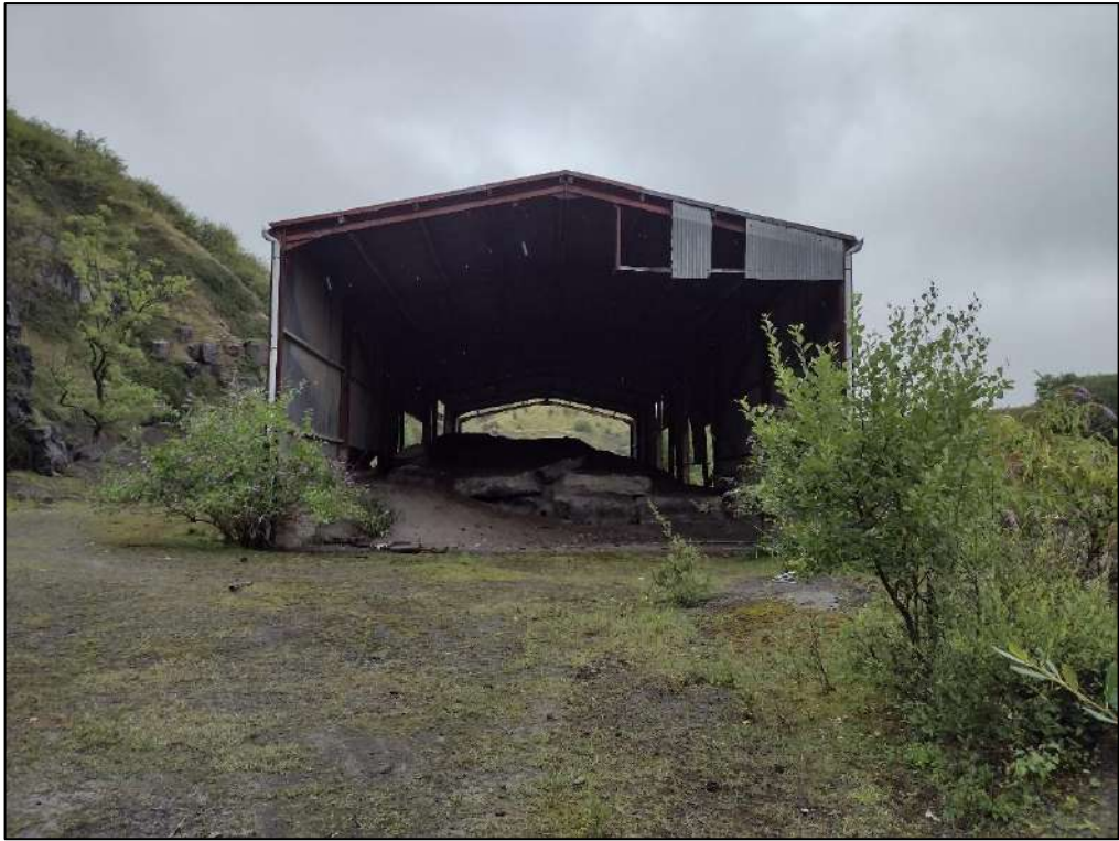
Photo 8. Storage building 1, south facing elevation
