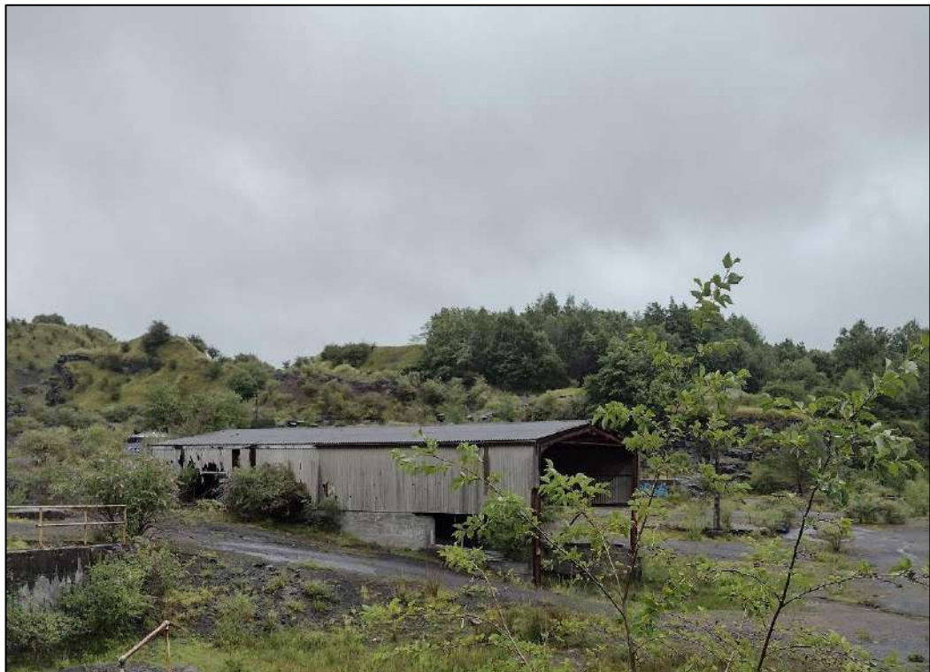
Photo 9. Storage building 2, west facing elevation
