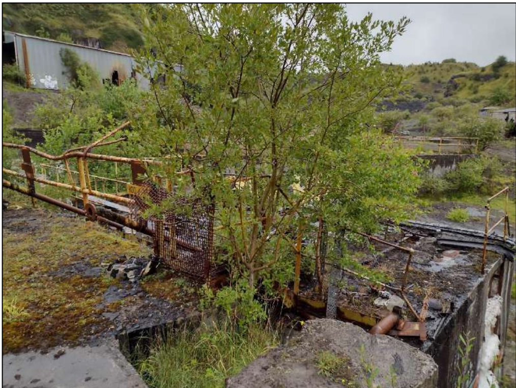
Photo 6. Remains of concrete structure 4 (Fig. 13, 6), looking north
