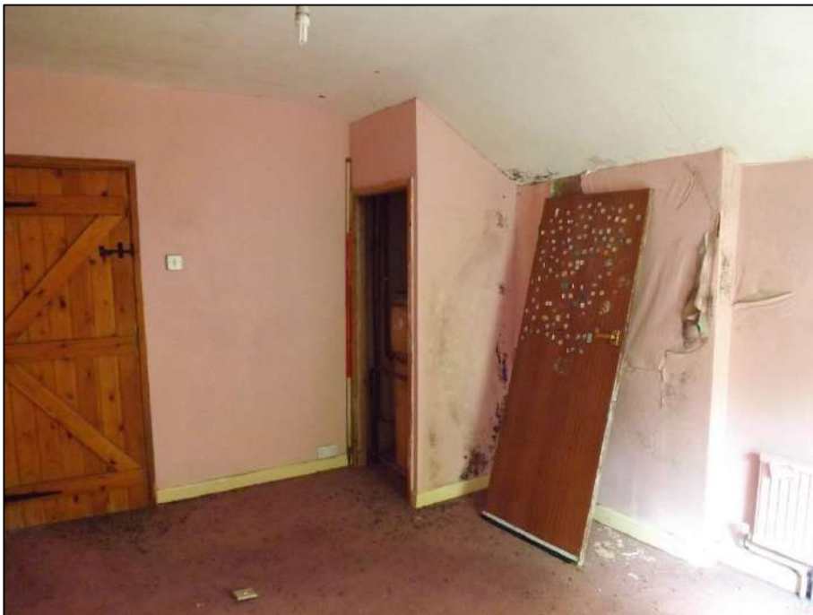
Plate 43. Plasterboard boiler cupboard within the south west bedroom. Note the childrens' stickers on the door, the only sign of personalisation within the entire cottage. Scale 2m.
