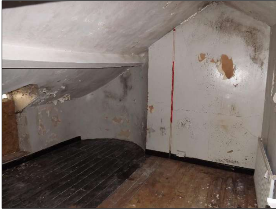
Plate 41. Semi-circular feature in the south east corner of the main bedroom. Note the cut line in the floorboards. This feature may be the vestigial remains of a stairwell. Scale 2m.
