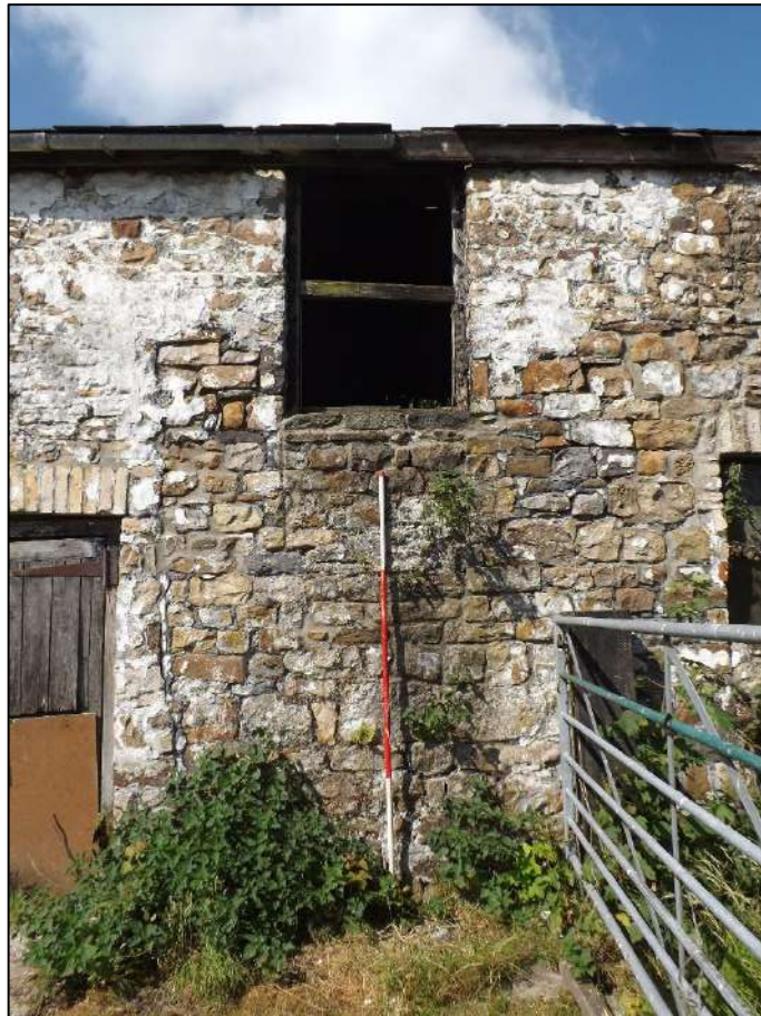
Plate 11. The northernmost upper window created by partially blocking a previous window or doorway, probably when the roofline was raised. Scale 2m.
