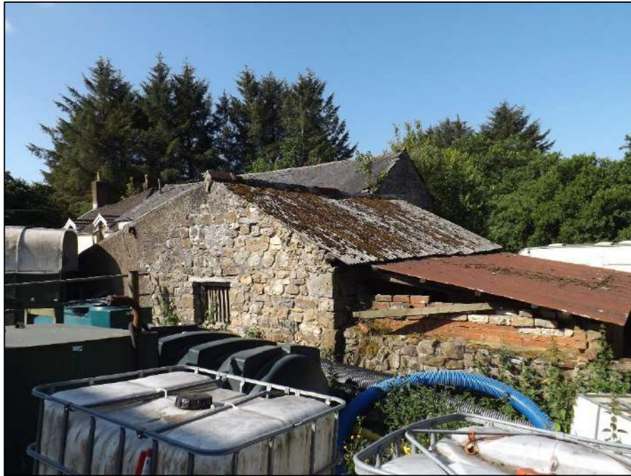
Plate 6. East elevation. Note the extension to the right of the image that shows how the old boundary wall has been utilised.
