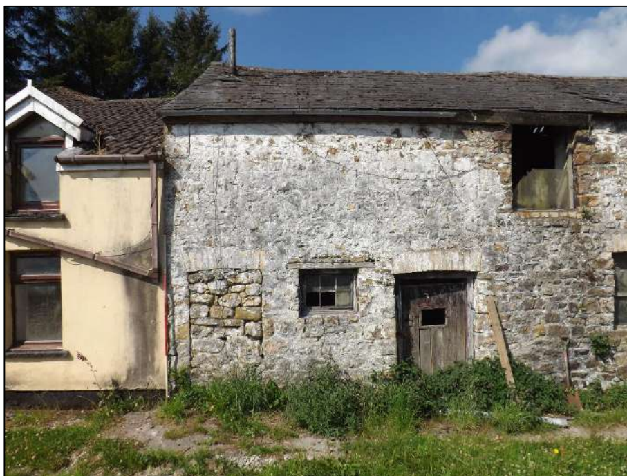
Plate 10. Southern end of the barn showing the blocked doorway. Scale 2m.
