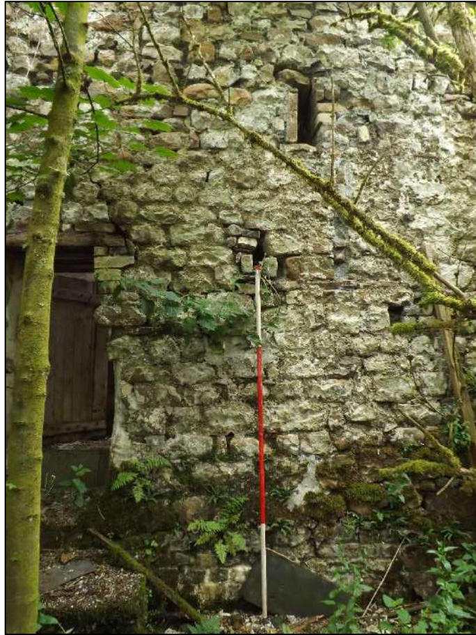
Plate 22. Detail of the west elevation on the barn showing possible air vent and possible scaffolding hole. Scale 2m.
