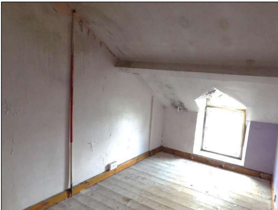
Plate 45. View into the north east bedroom showing dormer window arrangement and plasterboard ceilings.
