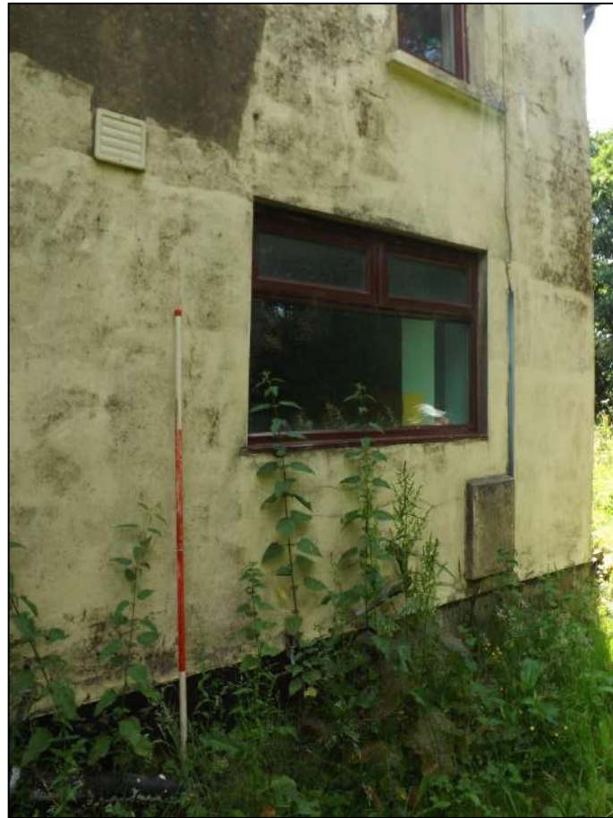
Plate 33. Ground floor kitchen window in the west elevation of the cottage. Scale 2m.
