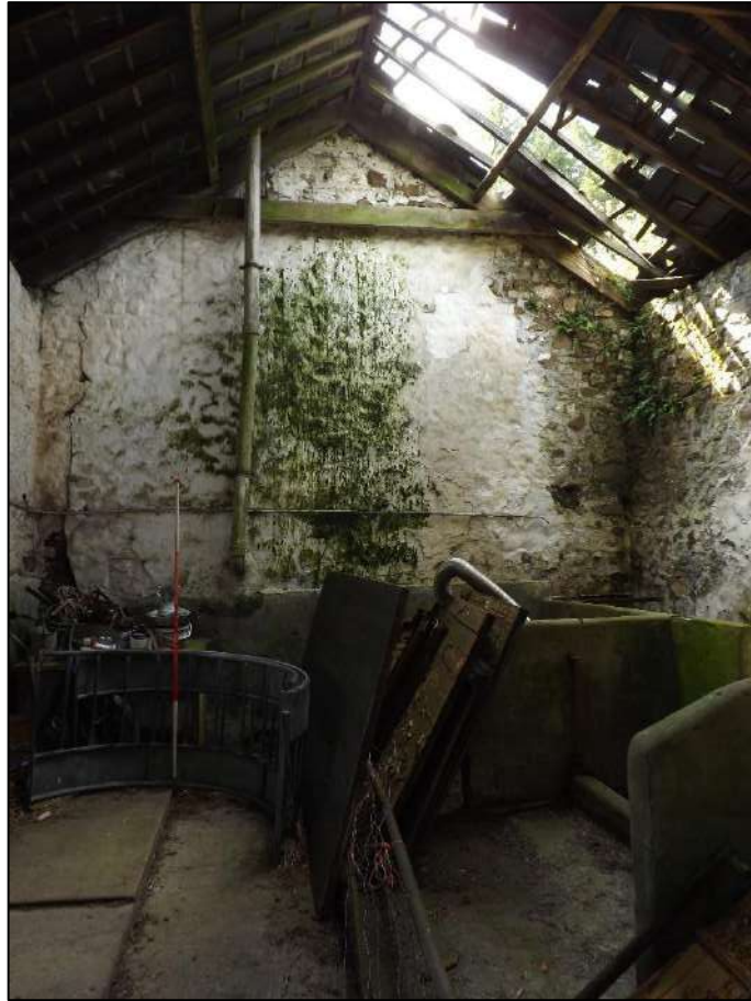
Plate 27. Interior of the south wall showing stored farm items and part of the byre. Scale 2m.
