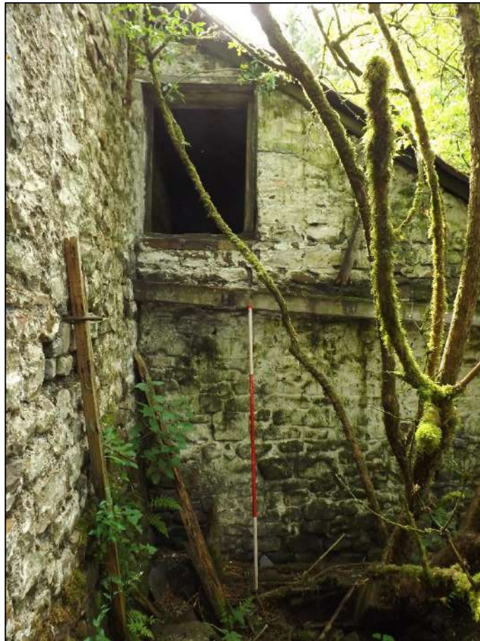
Plate 23. North elevation of Annexe 1 which also formed the south wall of Annexe 2. Note the window with surviving framing. Scale 2m.
