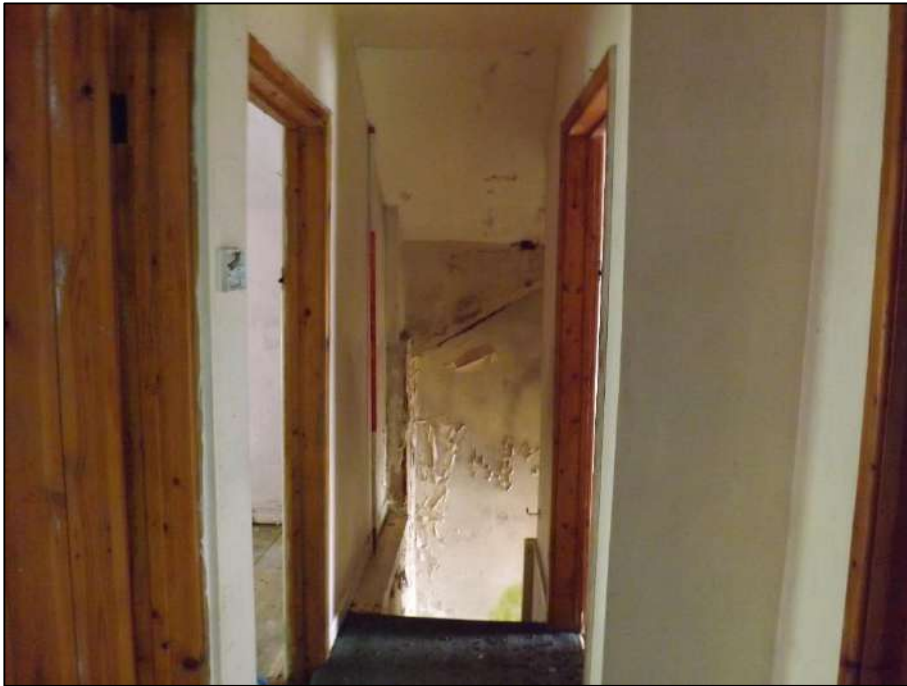
Plate 46. View along the landing towards the stairwell. Scale 2m.
