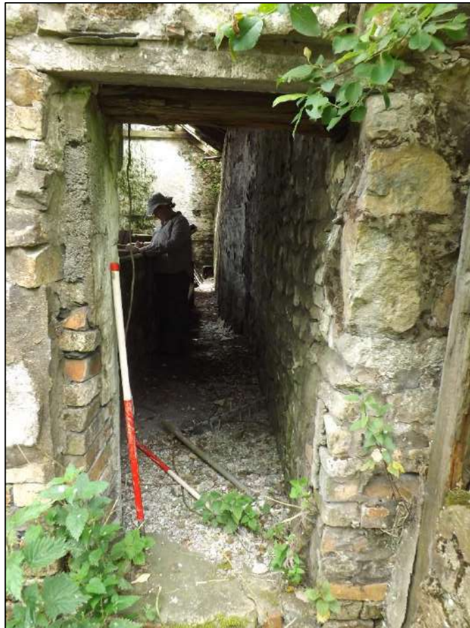
Plate 13. General picture of the doorway set into the north elevation of the barn. Note the breeze block and brick elements and the fact that there is no framing for a doorway. Scale 1m.
