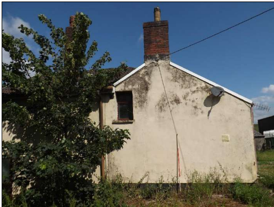
Plate 32. South elevation of the cottage. Scale 2m.
