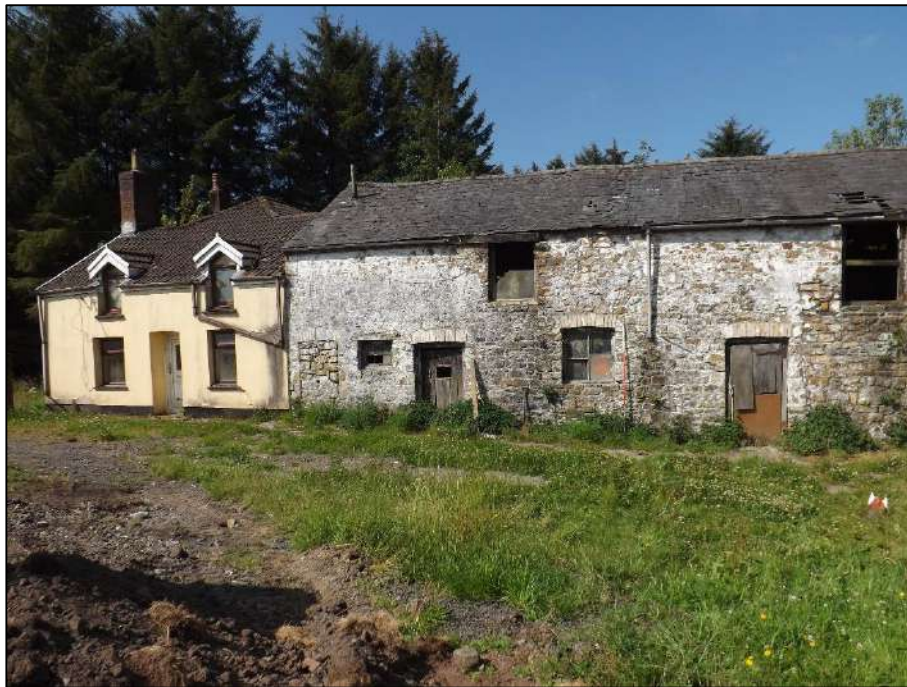
Plate 9. General view of the east elevations of both the barn (right) and cottage. Scale 2m.
