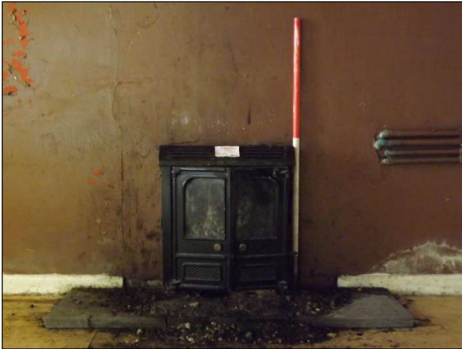
Plate 39. The fireplace in the living room. This is a later addition as fractures in the render and the gaps in the skirting board indicate the presence of an earlier fireplace behind the grate. Scale 1m.
