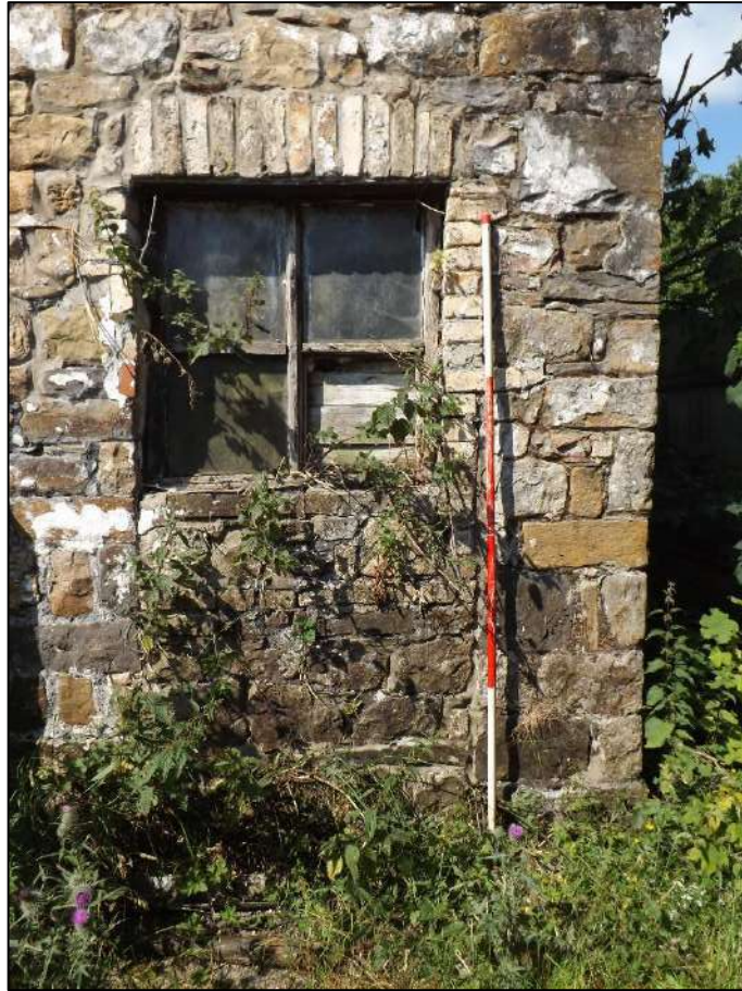
Plate 12. Blocked doorway at the north of the east elevation. Unlike the blocked doorway to the south, this was converted to a window. Scale 2m.
