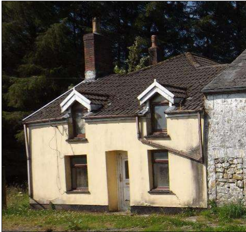
Plate 31. Oblique view of the east elevation of the cottage. No scale but the doorway measured 2m in height by 1m in width.
