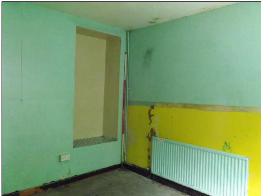
Plate 35. Rectangular recess in the south east corner of the kitchen. This was almost certainly a blocked doorway that once led into the barn that was repurposed for storage.
