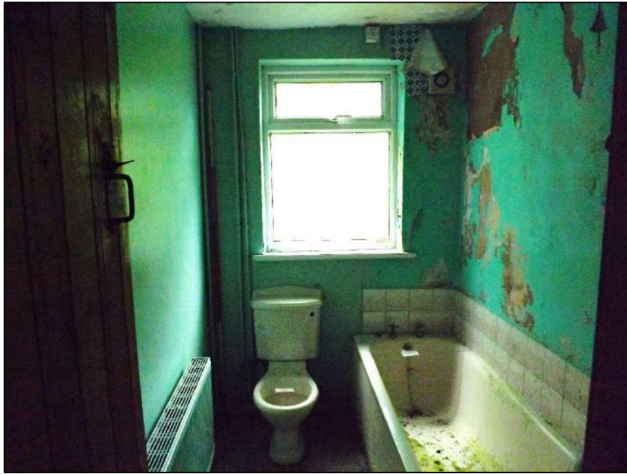
Plate 36. Modern bathroom on the ground floor. Scale to the left of the toilet 2m.
