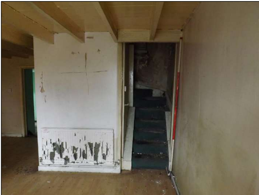
Plate 40. View of the stairwell leading to the first floor. Scale 2m.
