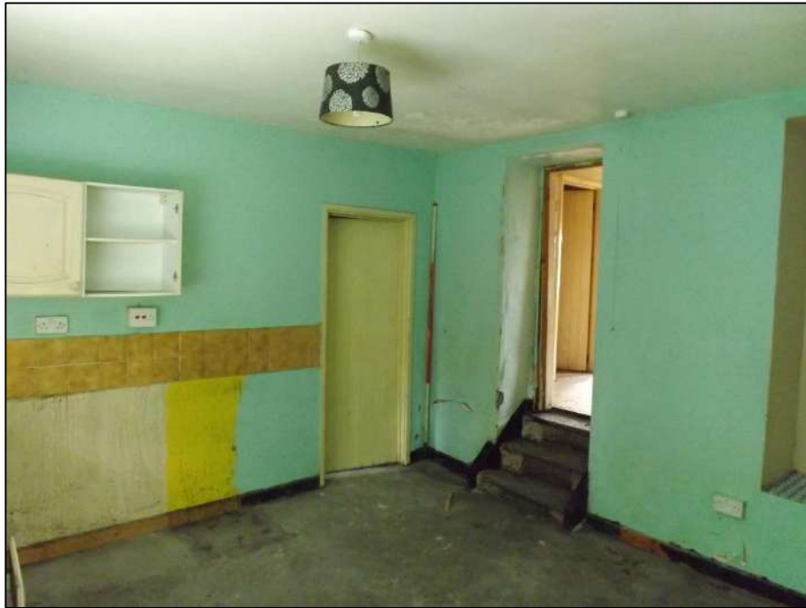
Plate 34. North east corner of the kitchen showing the steps into the living room and doorway (closed) into the bathroom. Scale 2m.
