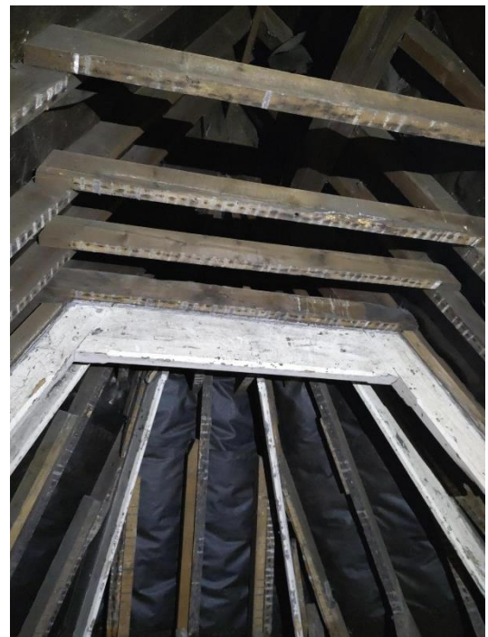
Figure 25 - Wooden beams on second floor.
