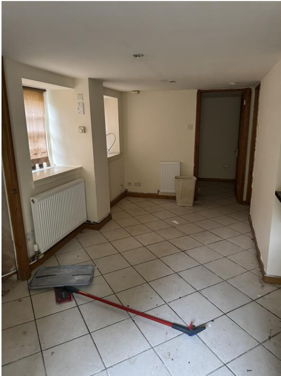
Figure 46 - Basement of Primrose Hill.
