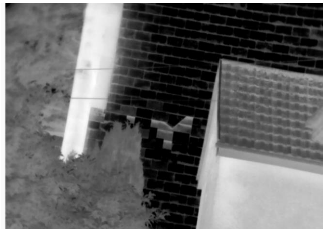
Figure 75 - Bat Survey 2 FLIR NVA (South Aspect of Roof) 17/07/2024.
