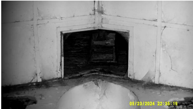
Figure 70 - Bat Survey 1 IR NVA (Internal Camera, Loft Hatch) 23/05/2024.
