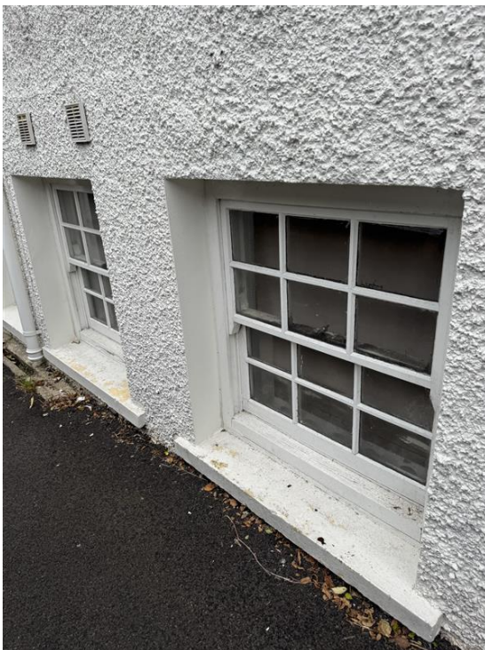
Figure 48 - Windows of Primrose Hill basement flat.
