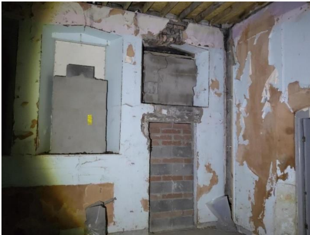
Figure 8 - Exposed brickwork on the ground floor.
