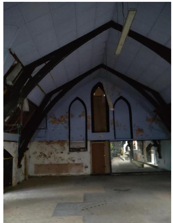
Figure 29 - Internal space on second floor.
