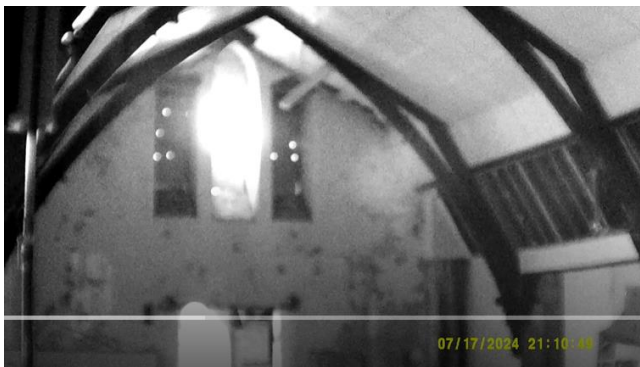
Figure 74 - Bat Survey 2 IR NVA (West Aspect) Internal Camera 17/07/2024.
