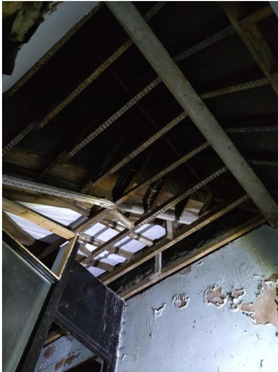
Figure 22 - Wooden beams on second floor.
