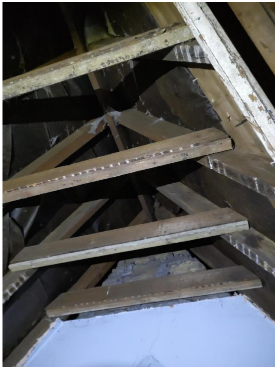
Figure 28 - Wooden beams on second floor.
