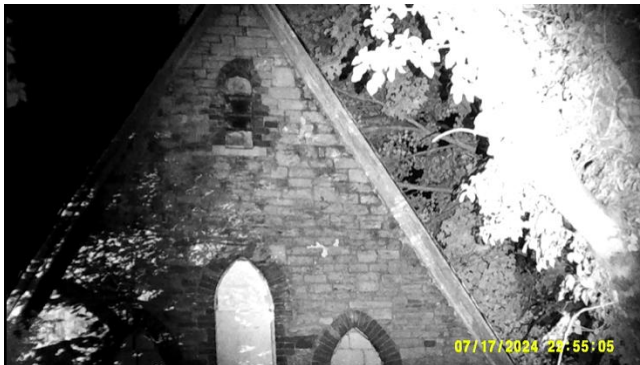
Figure 72 - Bat Survey 2 IR NVA (East Aspect) 17/07/2024.
