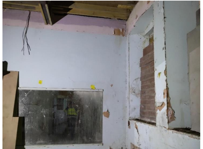
Figure 11 - Bricked up windows on ground floor.
