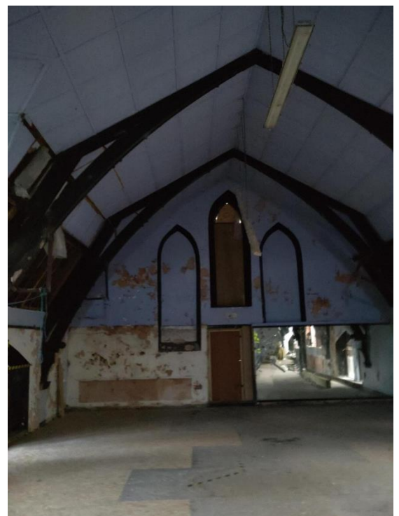
Figure 29 - Internal space on second floor.
