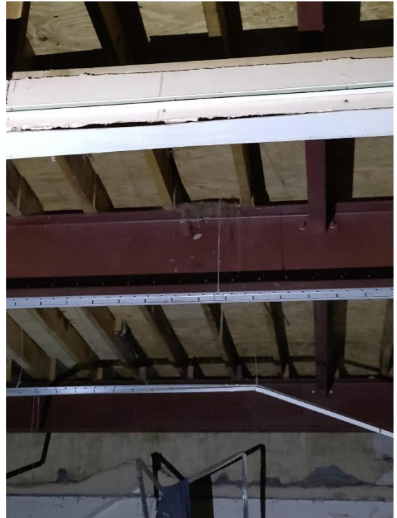
Figure 23 - Wooden beams on second floor.
