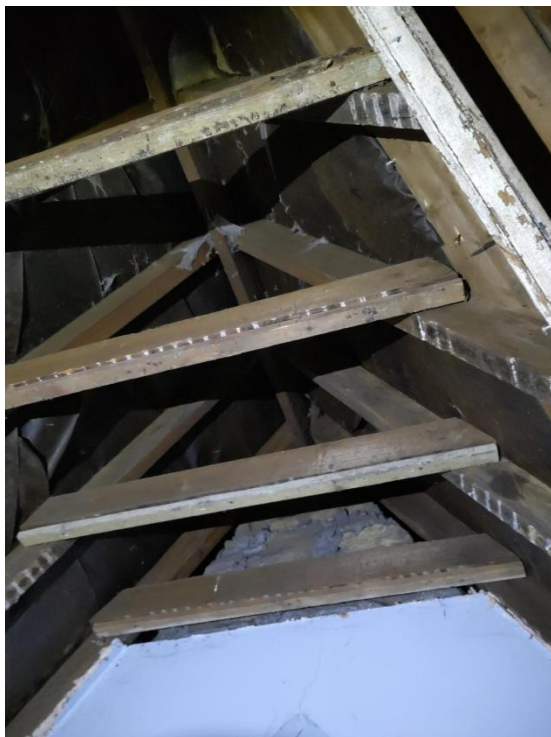
Figure 28 - Wooden beams on second floor.
