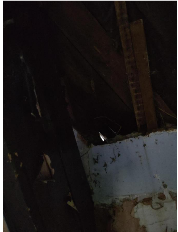
Figure 31 - Gaps in roofing felt on second floor.
