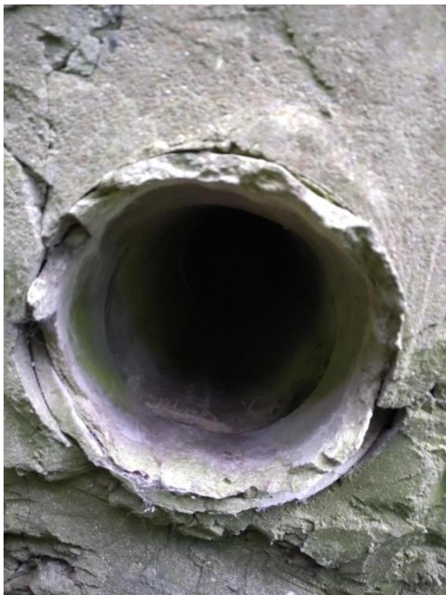
Figure 36 - Pipe on northern aspect of building.
