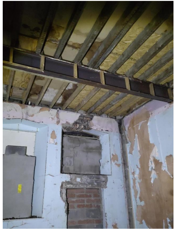
Figure 15 - Exposed brickwork on ground floor.
