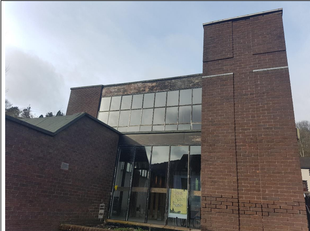
Photo 1. East elevation and tower
