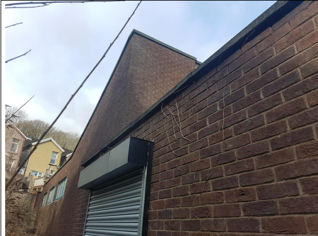
Photo 4. South elevation including new shutter over kitchen window
