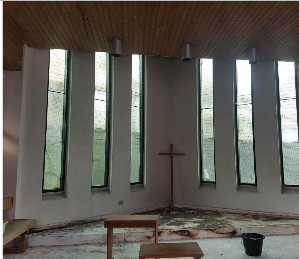
Photo 9. Interior looking west showing wood clad ceilings
