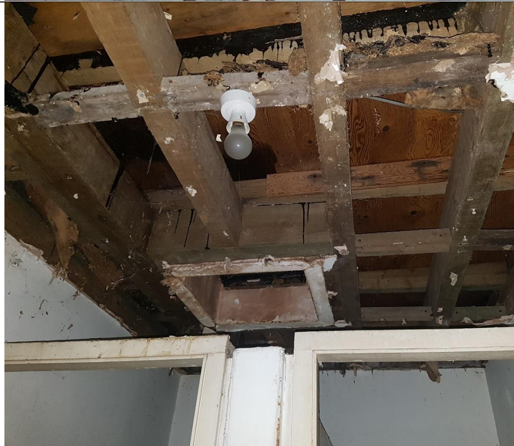
Photo 10. Ceilings removed in the toilets
