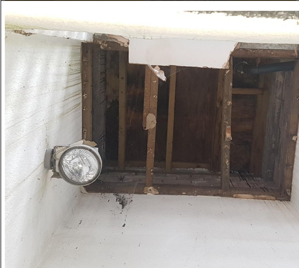
Photo 12. Ceiling removed inside tower
