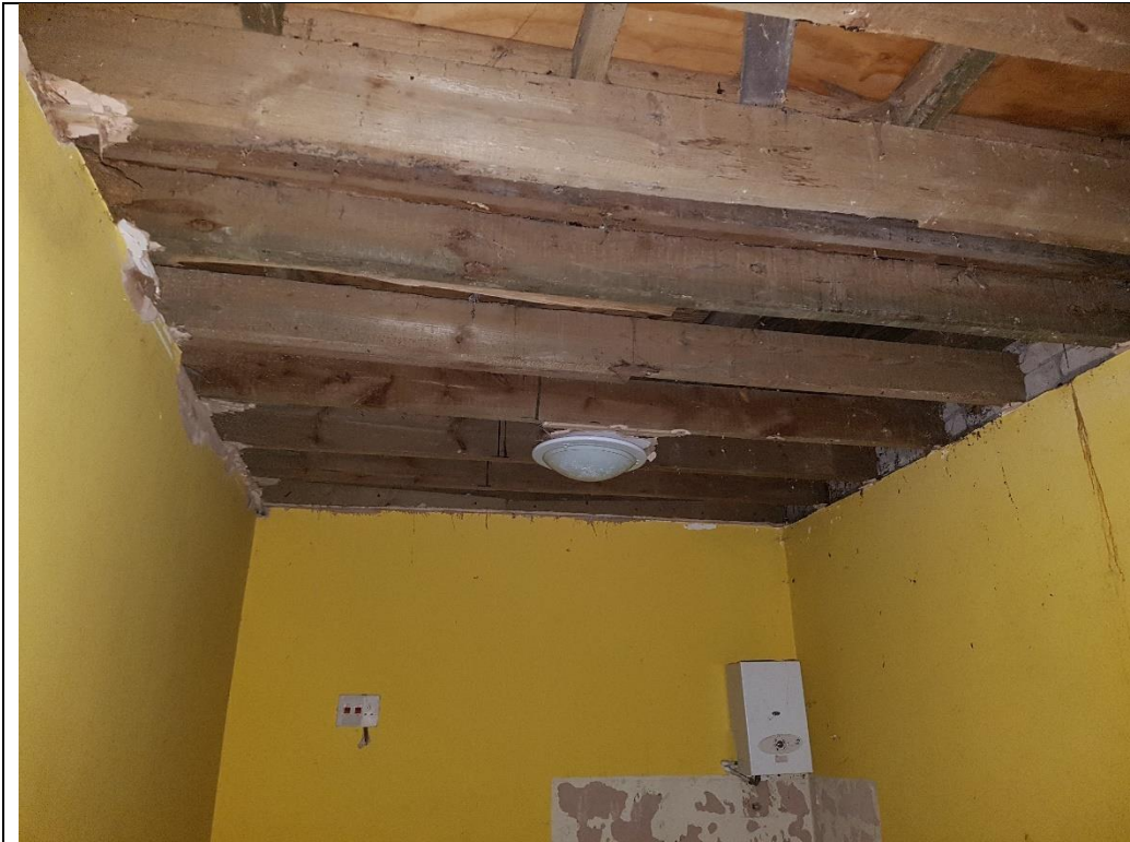
Photo 11. Ceiling removed in the former kitchen
