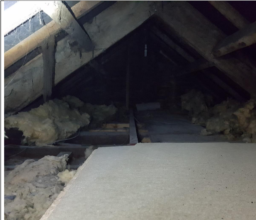
Photo 8 General view inside main cottage loft
