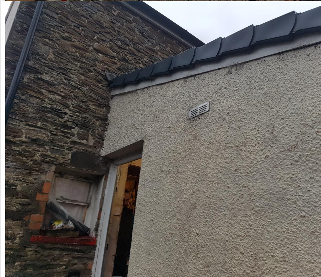
Photo 3. Side of extensio n (north)
