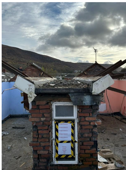
Figure 4: The soft strip and roof removal was completed.
