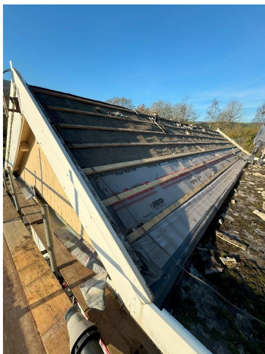
Figure 3: All tiles removed.
