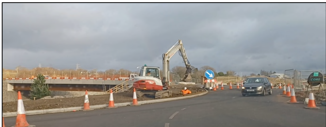
Plate 3.3 Prince Charles Hospital Junction – eastern overbridge looking North from Gurnos Ring Road (start of February 2025)
