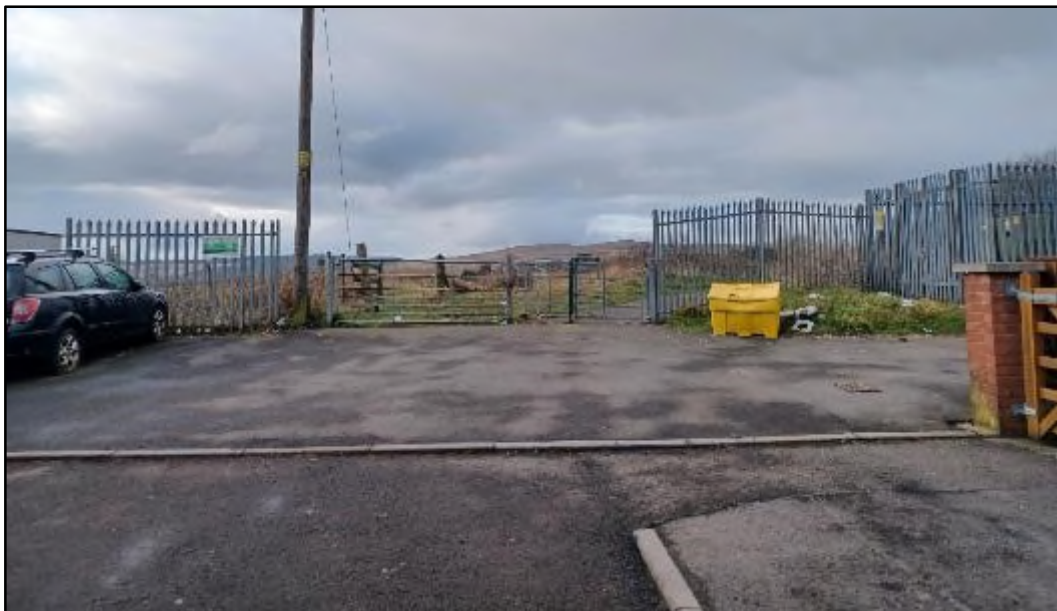
Plate 3.1 Existing access looking west from Sixth Avenue
