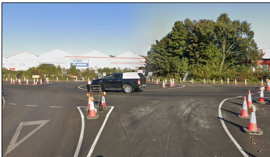
Plate 3.2 A465 Heads of the Valleys Road Temporary Roundabout Junction with Rocky Road (start of February 2025)
