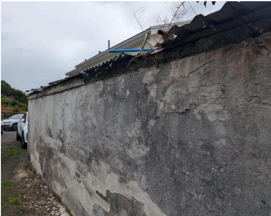
Plate 2- example of fascia and damage
