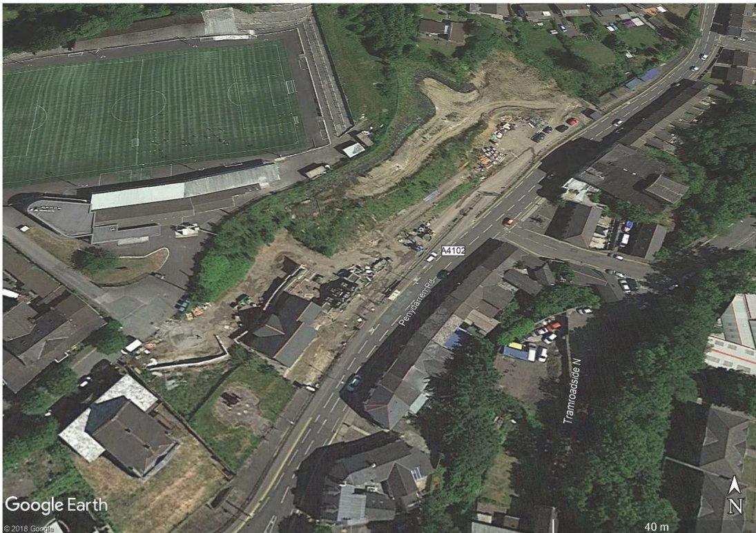
Aerial view of the site with adjacent residential development in progress
