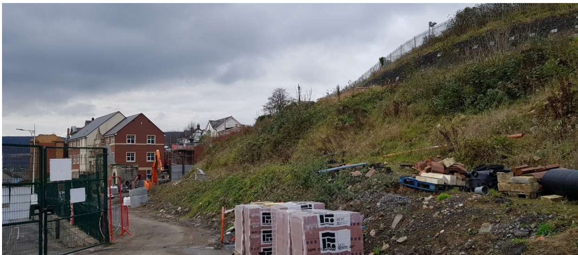
View west towards new residential development (prior to slope reinstatement)
