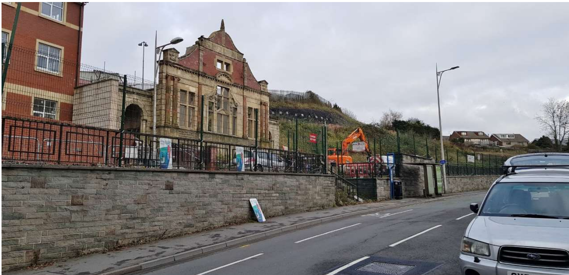
View north with new residential development on far left (prior to slope reinstatement)
