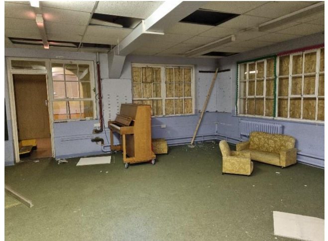
Figure 4 – Another typical view inside a room.
