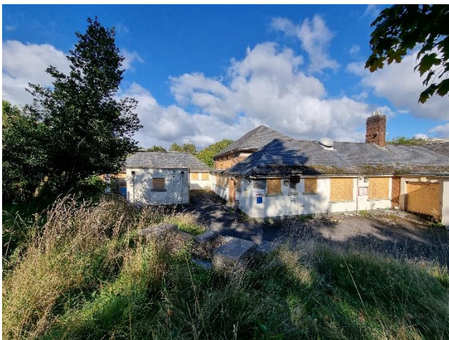
Figure 11 – View across the building, looking north-east.
