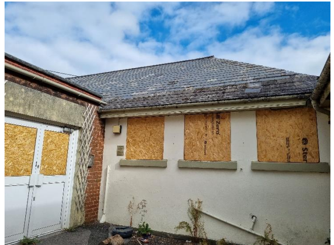
Figure 6 – Building main entrance.
