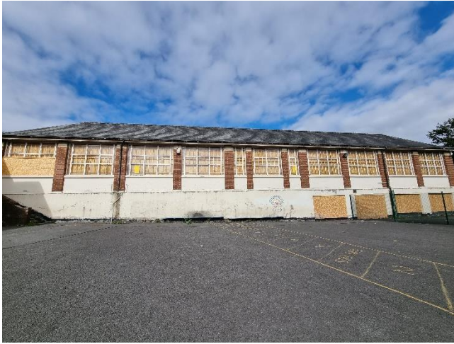
Figure 7 – North-west section of building.
