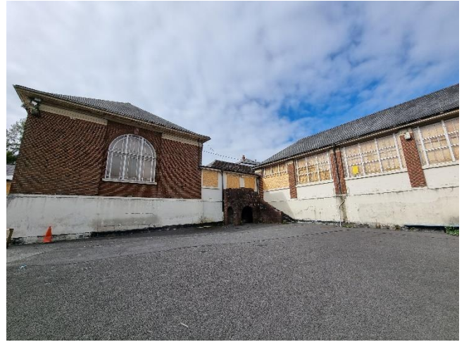
Figure 8 – Looking south towards the centre of the building.
