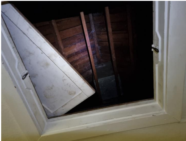
Figure 5 – Attic access was usually left open but not accessed due to damp concerns.
