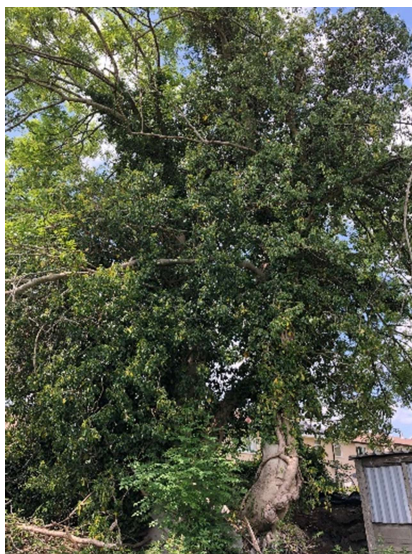
Figure 4 Ivy covered ash
