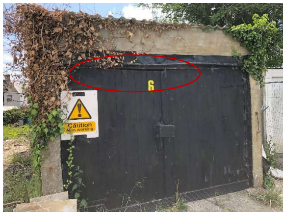
Figure 2 Garage building with potential access point above door
