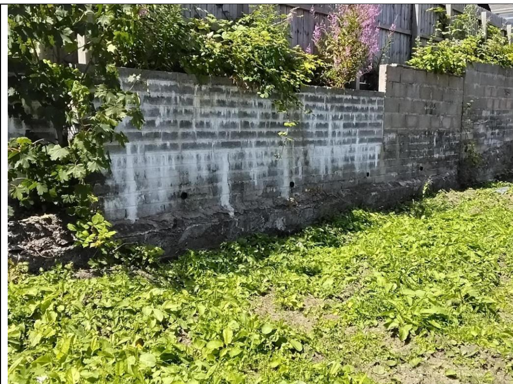
East boundary, block wall
