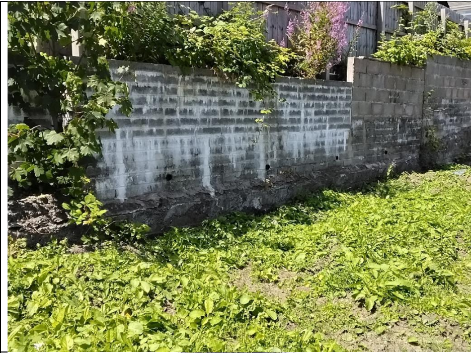
Photo 5. Block wall making up the west boundary
