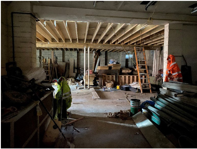
Figure 9 – internal view of lower ground floor
