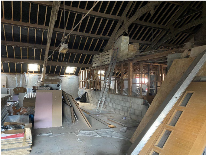
Figure 7 – internal view of upper ground floor showing open nature of internal space, timber work and breathable membrane installed
