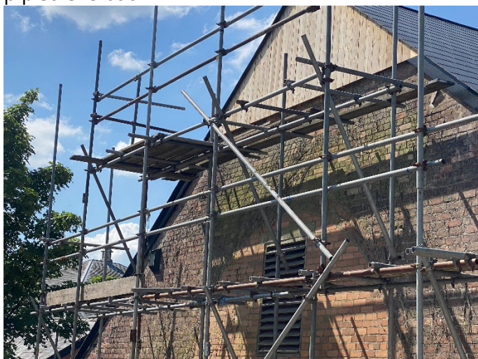
Figure 5 – cladding mitigation in closer detail and bat box on northeast elevation
