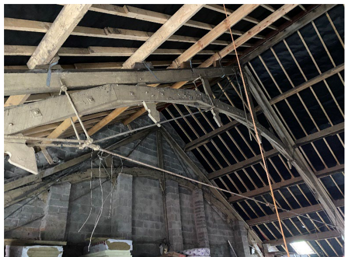
Figure 6 – internal view of upper ground floor showing open nature of internal space, timber work and breathable membrane installed
