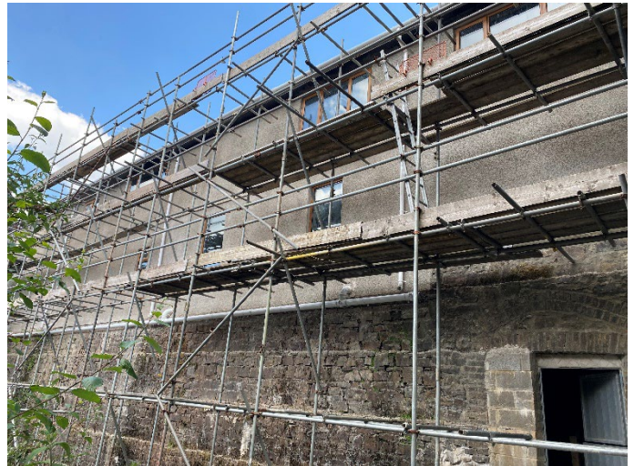
Figure 4 – east elevation adjacent to Nant Morlais and basement door
