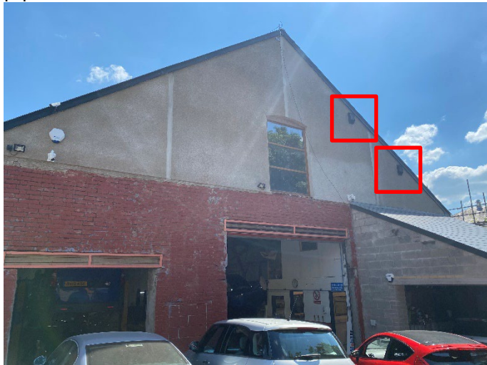
Figure 3 – southwest elevation and gable end with 2 x bat boxes as bat roost mitigation for pipistrelle bat
