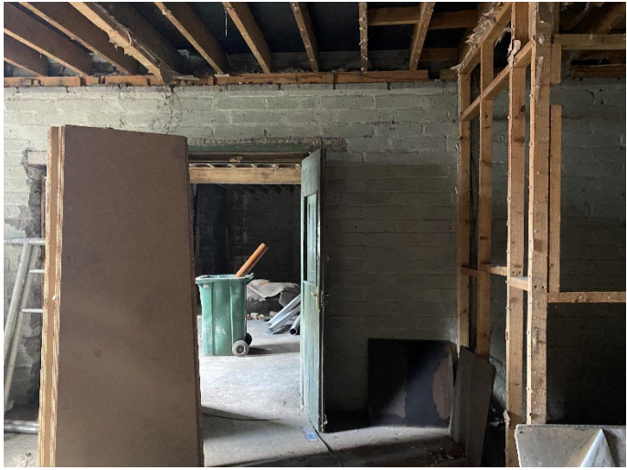
Figure 8 – internal view of lower ground floor
