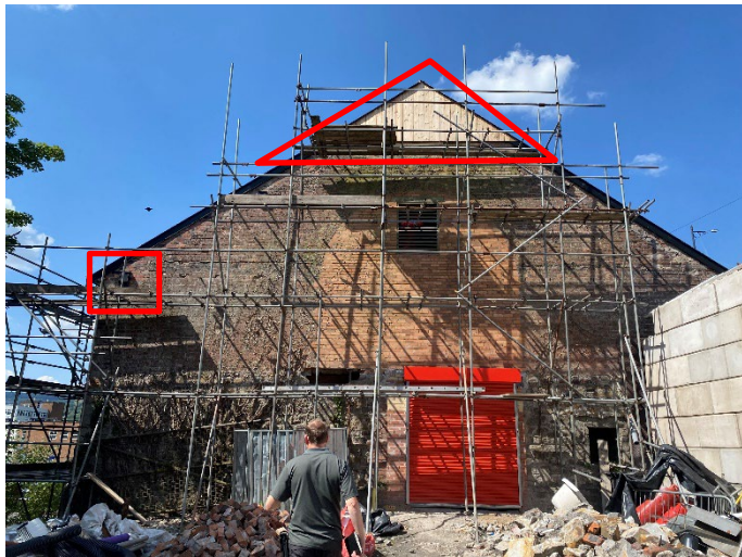
Figure 1 – northeast elevation and gable end with timber cladding provided as bat roost mitigation for long-eared bat and a single bat box for pipistrelle bat
