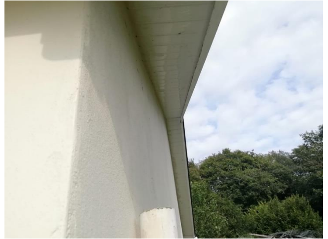
Figure 4 – Southern gable of garage with tightly sealed soffit
