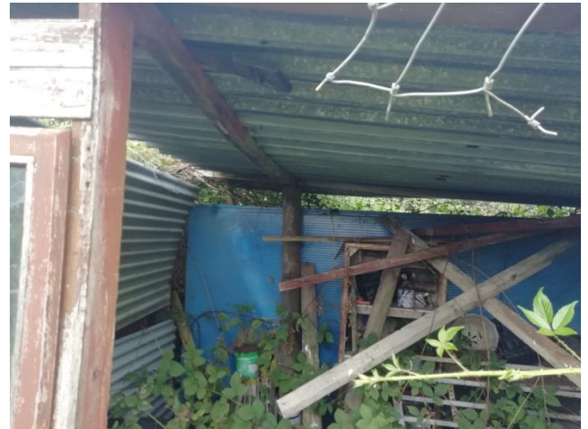
Figure 16 – Interior of second outbuilding
