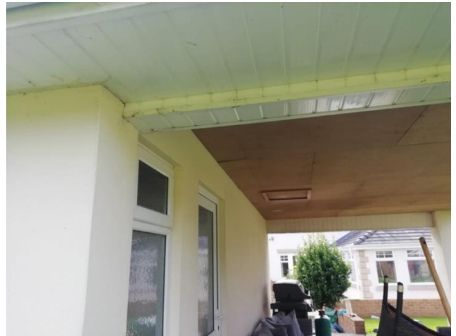
Figure 10 – Underside of sheltered area (northern section)
