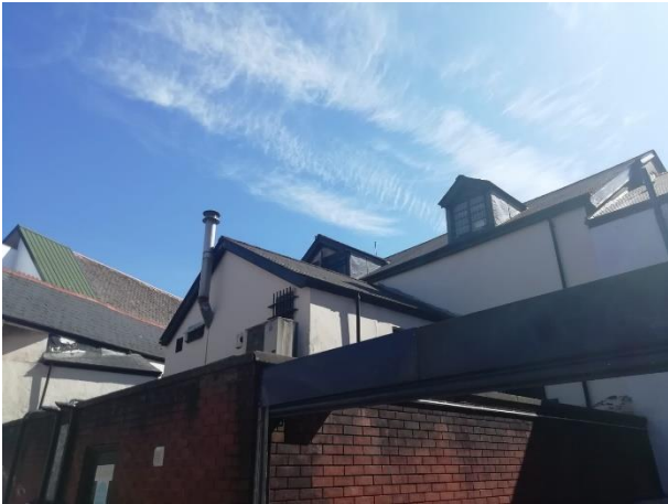
Figure 6 – View of rear of building looking towards south-east
