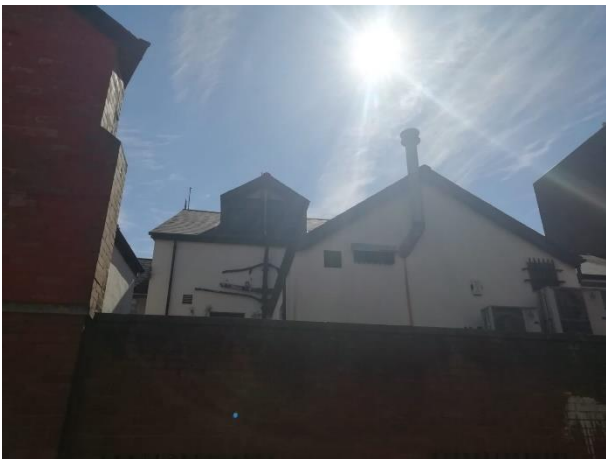
Figure 7– View of rear of building looking towards south
