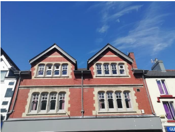
Figure 5 – View of front (southern aspect) of building
