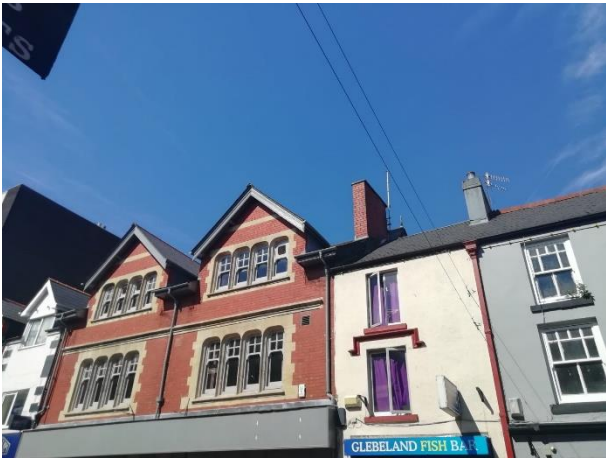
Figure 4 – View of front of building (from opposite side of street) with partial view of roof (eastern parts)
