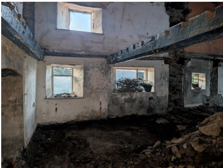
Plate 5 - Gutted ground-floor room showing multiple small window openings, exposed bressummer/ceiling beams and a bare earth and rubble floor.
