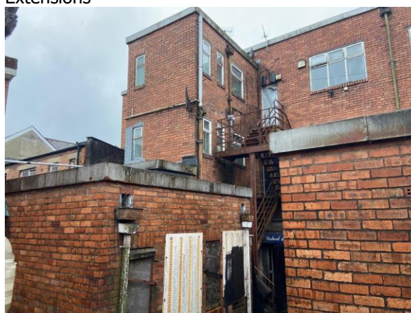
Photo 2: Eastern Rear Showing Single-storey Extensions
