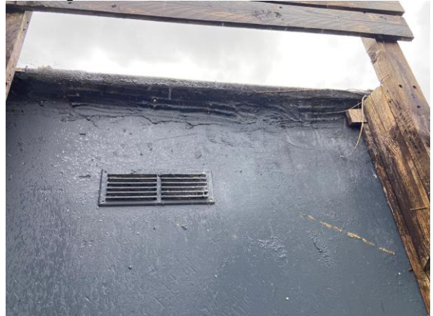
Photo 6: Easternmost Single-storey Extension Showing Vent and Bitumen Felt Roof
