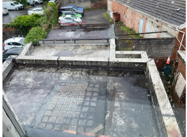
Photo 6: Easternmost Single-storey Extension Showing Vent and Bitumen Felt Roof
