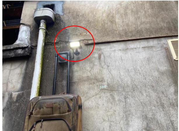
Photo 12: Security Light at the Rear (Circled)
