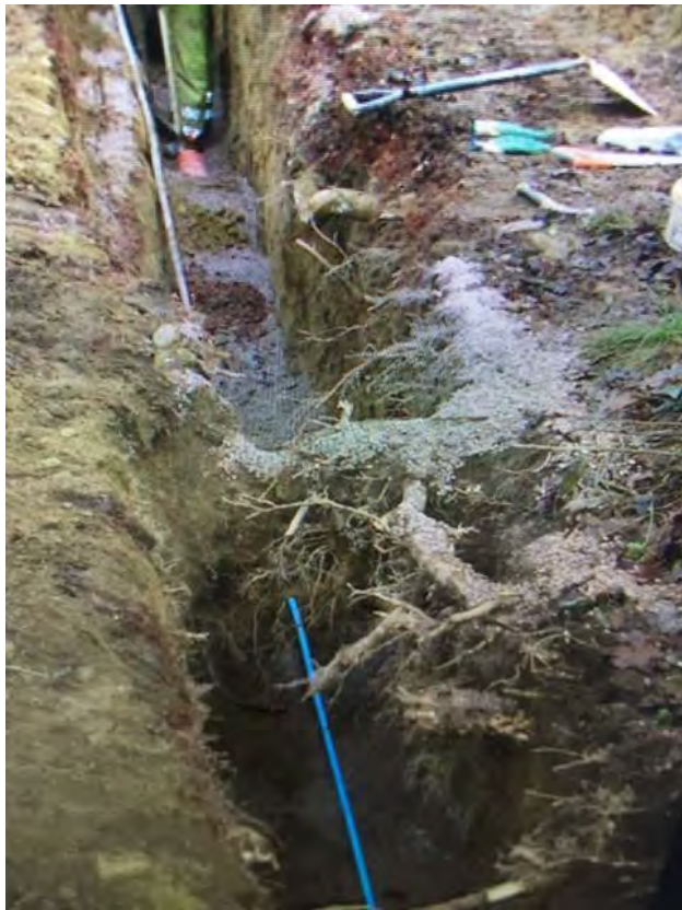
The above photo shows how narrow, hand-dug trenches can be used to route services through sensitive parts of woodland without affecting existing trees. When determining the route of a trench, care is taken to understand the local environmental conditions as this can have a bearing on the way that roots grow underground which anchor the tree against prevailing winds. Service routes as those above will ensure that the disturbance of local soil will not weaken the structural integrity of the tree in its surrounding soil
