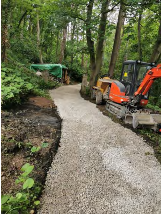
Typical new track construction. The photos show examples of how typical tracks will look immediately upon completion. Note that the areas alongside the track is constructed of banked earth and will be colonised with native undergrowth over the subsequent growing season.
