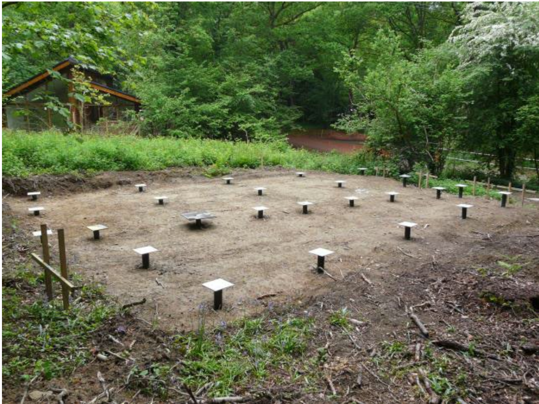
Figure EDP 5.1: Piles for platform of lodges (©Holder Mathias).
