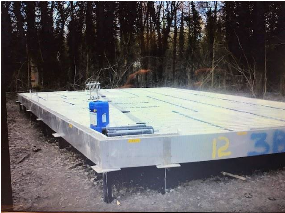
Figure EDP 5.2 Raised lodge platform on piles (©Holder Mathias).
