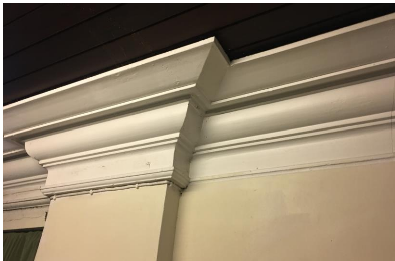
Existing cornice to number 20 to be retained
