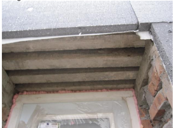
Plate 16: Gaps at exposed lintels, where care must be taken when sealing them off
