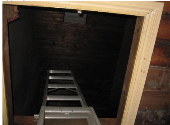
Plate 8: Western loft with timber sarking, entrance obstructed by partly fixed ladder
