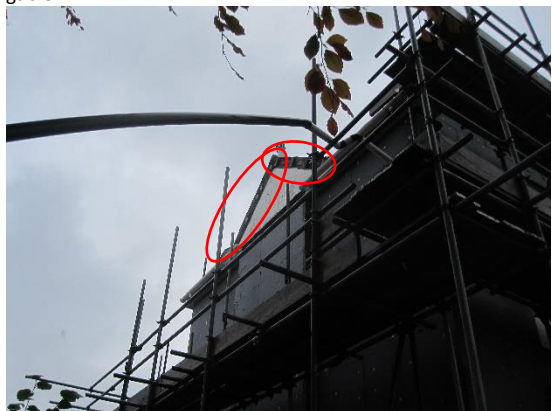
Plate 16: Gaps at exposed lintels, where care must be taken when sealing them off
