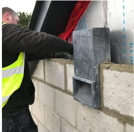
Plate 18: Example of integrated box being put in place
