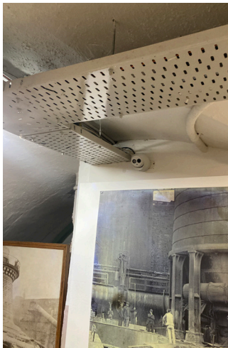
Cable trays run around the majority of the basement spaces to feed existing cameras and will be used for the majority of new camera locations..
