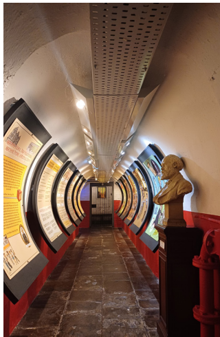
Cable trays run around the majority of the basement spaces to feed existing cameras and will be used for the majority of new camera locations..
