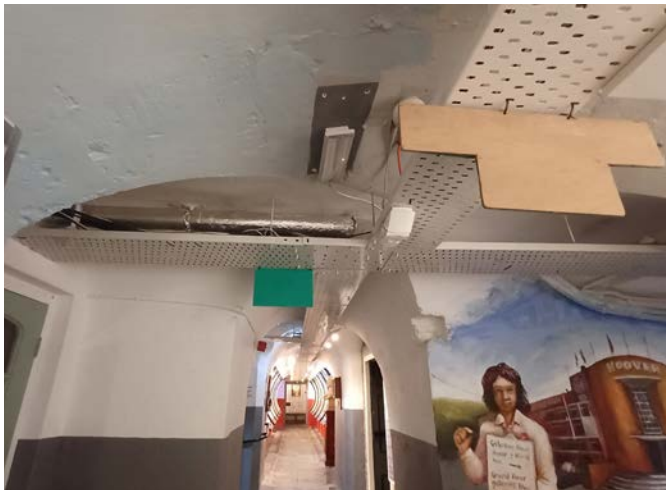
Cable trays run around the majority of the basement spaces to feed existing cameras and will be used for the majority of new camera locations..
