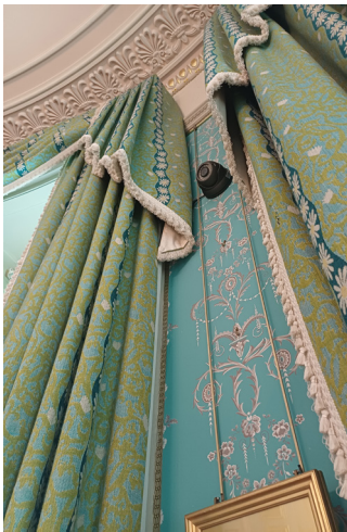
Example of trunking which is installed alongside architraves and concealed behind curtains.
