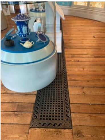
Cabling to be run in floor grilles.
