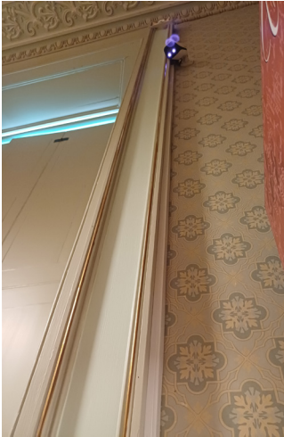
Examples of trunking which is installed alongside architraves resulting in a discrete finish.
