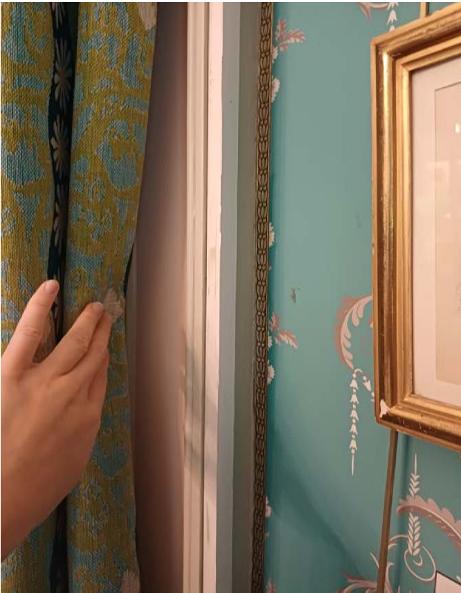
Painted trunking at window architrave to be reused
