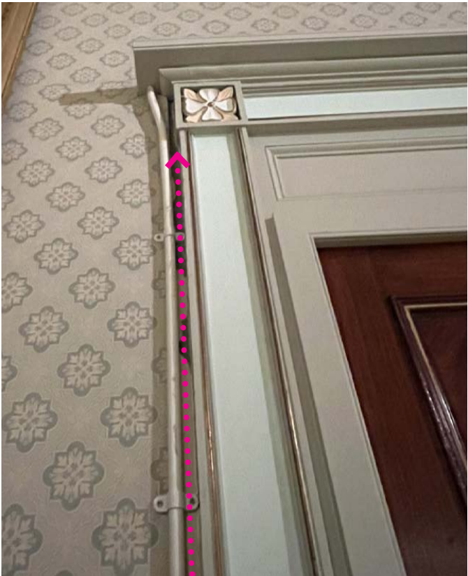
F1 - new micro trunking fits in gap between existing circular trunking and door architrave
