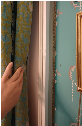
Example of trunking which is installed alongside architraves and concealed behind curtains.
