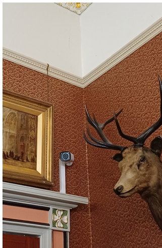
Example of locations where trunking is to be wall mounted. Trunking will be covered with wallpaper or painted in same colour as wall
