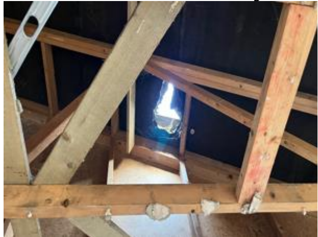
Photo 18: Tear in Bitumen Felt Roof Lining
