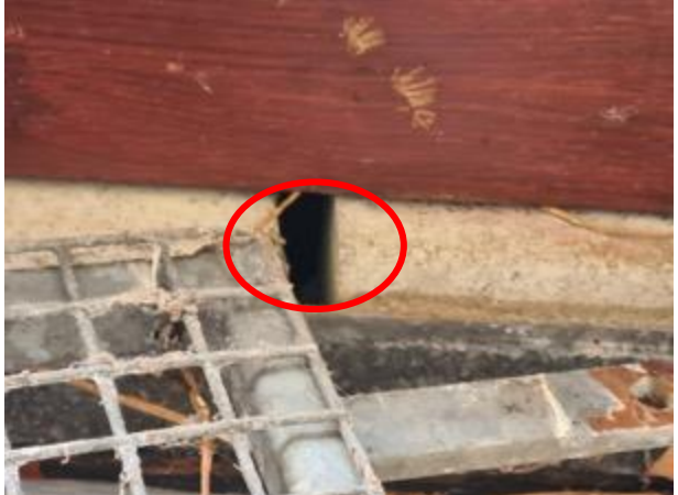
Photo 10: Gap Between Brick with the Missing Mortar, Above Window, Circled
