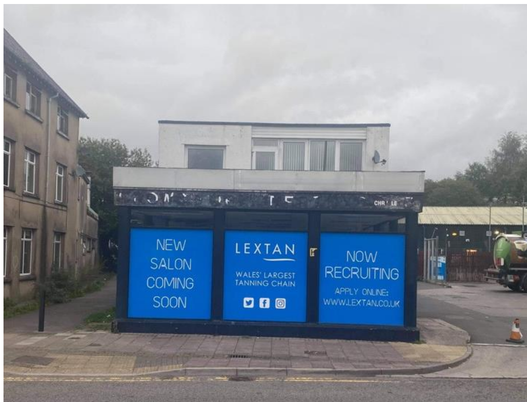
Fig. 2 – Front elevation of Unit 2
