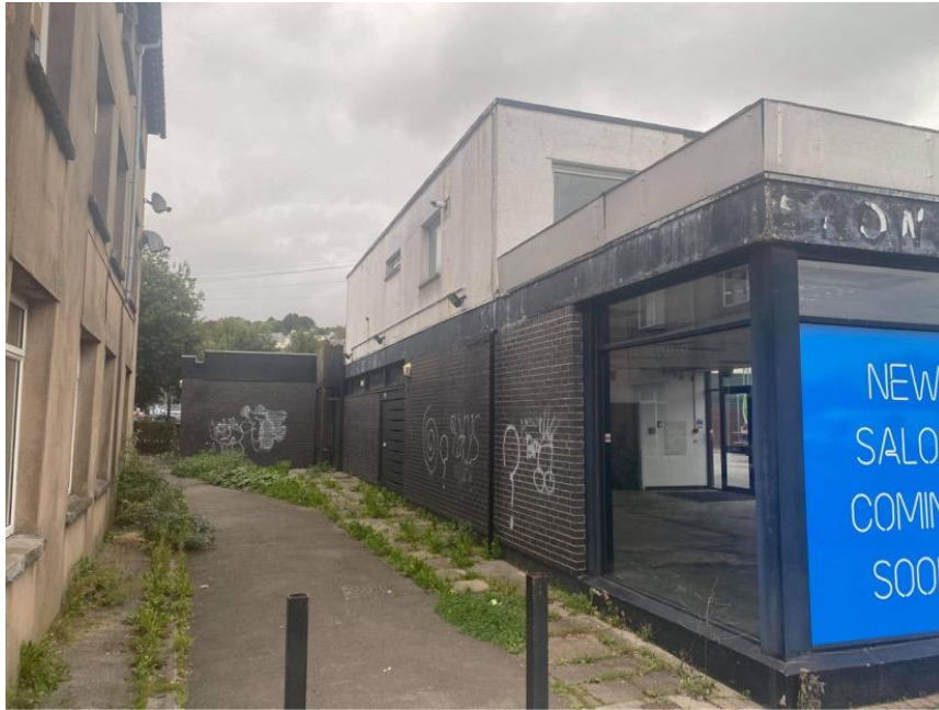
Fig. 3 – Side elevation of Unit 2 – Ex-servicemen's club on left
