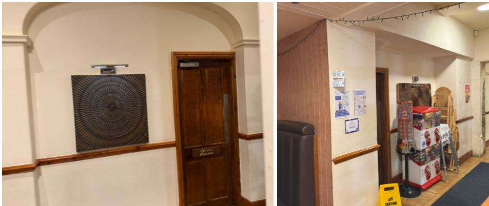
Figure 7.4 Modern infill walls to arch at Gent and wall to Ladies to be removed and new carvery area.
