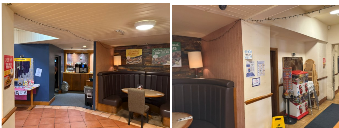
Figure 7.8 Modern walls and structures removed to allow carvery station
