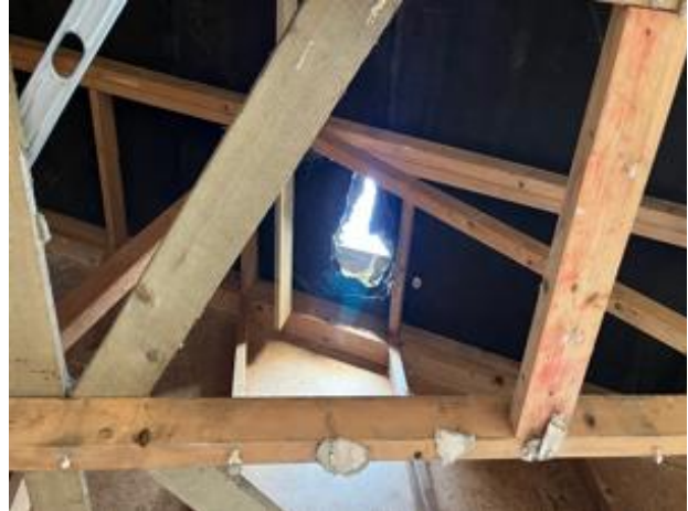
Photo 18: Tear in Bitumen Felt Roof Lining
