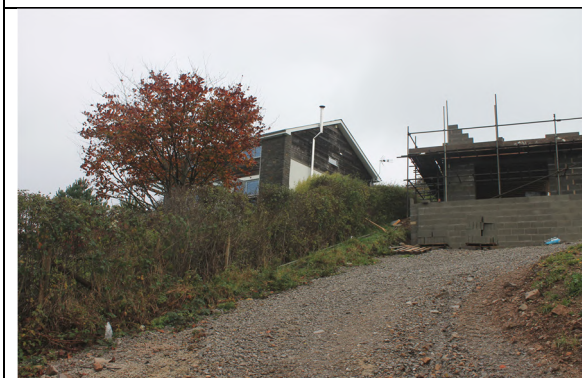
West boundary hawthorn hedge looking north
