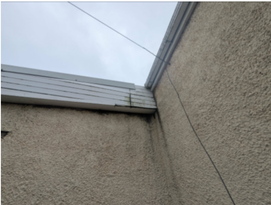
Plate 2- photograph of sealed fascias and soffits
