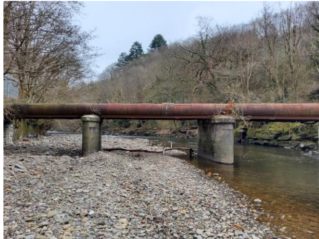
Photograph 1 View of feeder pipe bridge looking north upstream.
