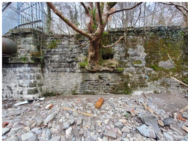
Photograph 4 Area of stone wall at north-west end of feeder pipe bridge. Gaps in walls suitable for bats to use for roosting.
