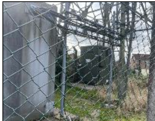
View through fence of buildings
