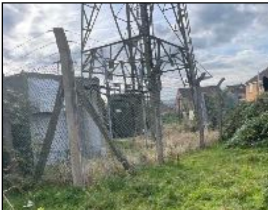
View of buildings and mast
