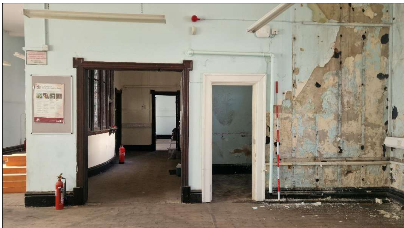
Plate 35. Wide opening to the reception and doorway to the former kitchen from the northern part of the Library, view to the south, 2m scale.
