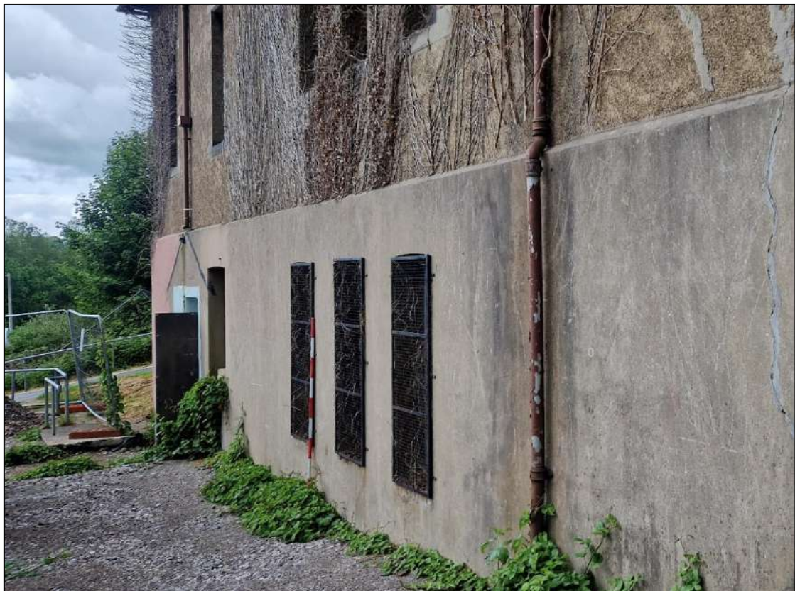
Plate 10. Rear elevation showing the basement level windows, view to the south-west, 2m scale
