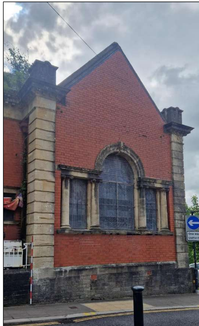
Plate 6. Southern bay of the front elevation, view to the south-east , 2m scale
