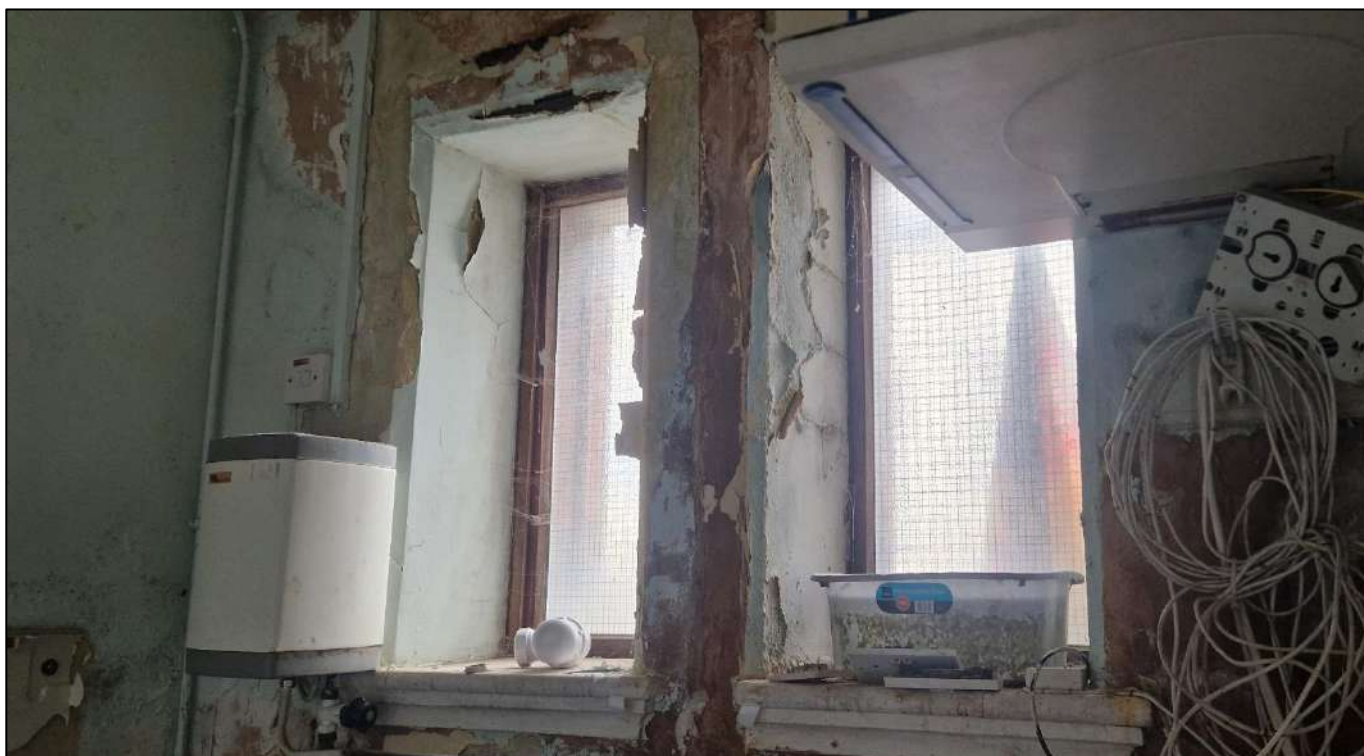
Plate 36. Windows within the former kitchen, view to the south-west.
