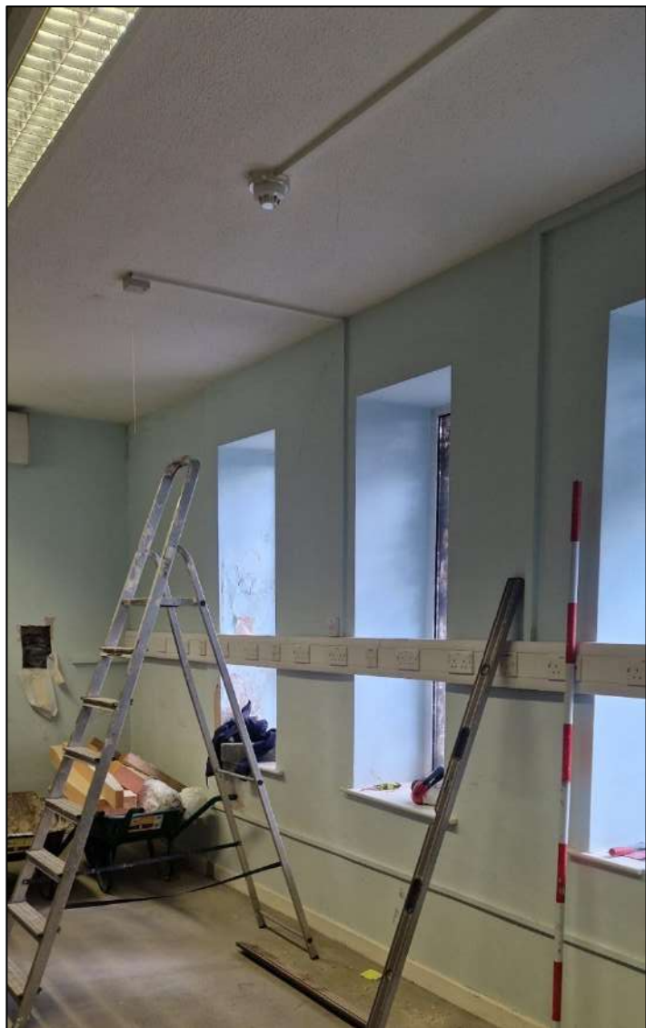
Plate 52. Windows in the Open Learning Room, view to the north-east, 2m scale.
