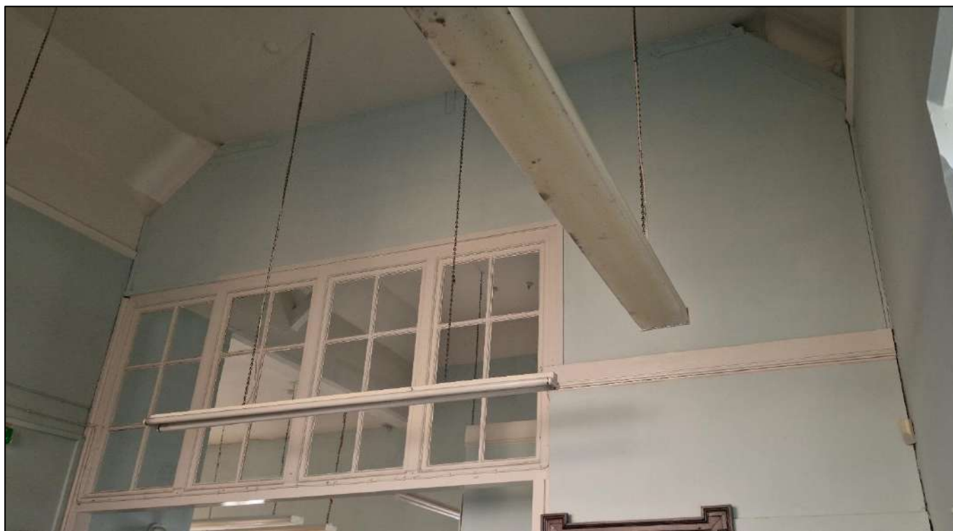
Plate 28. Upper section of the partition separating the Main Library from the Junior Library, view to the east
