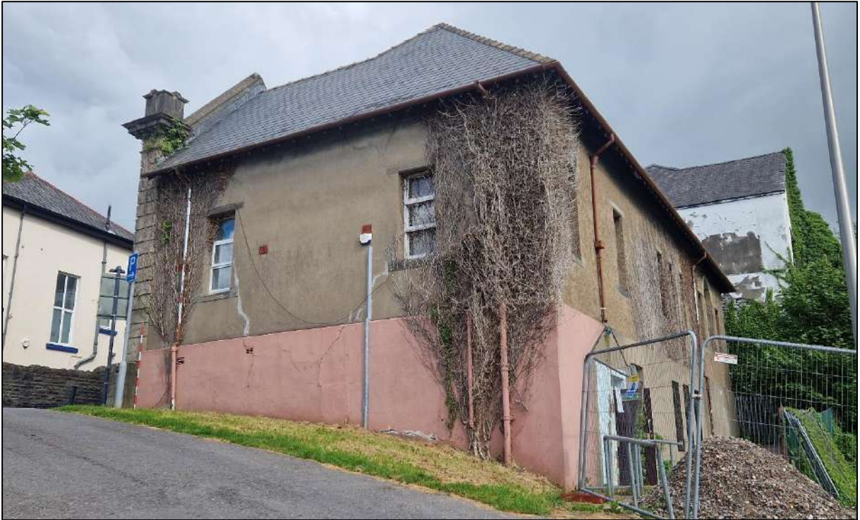
Plate 7. South elevation, following demolition of the extension, view to the north-west, 2m scale.
