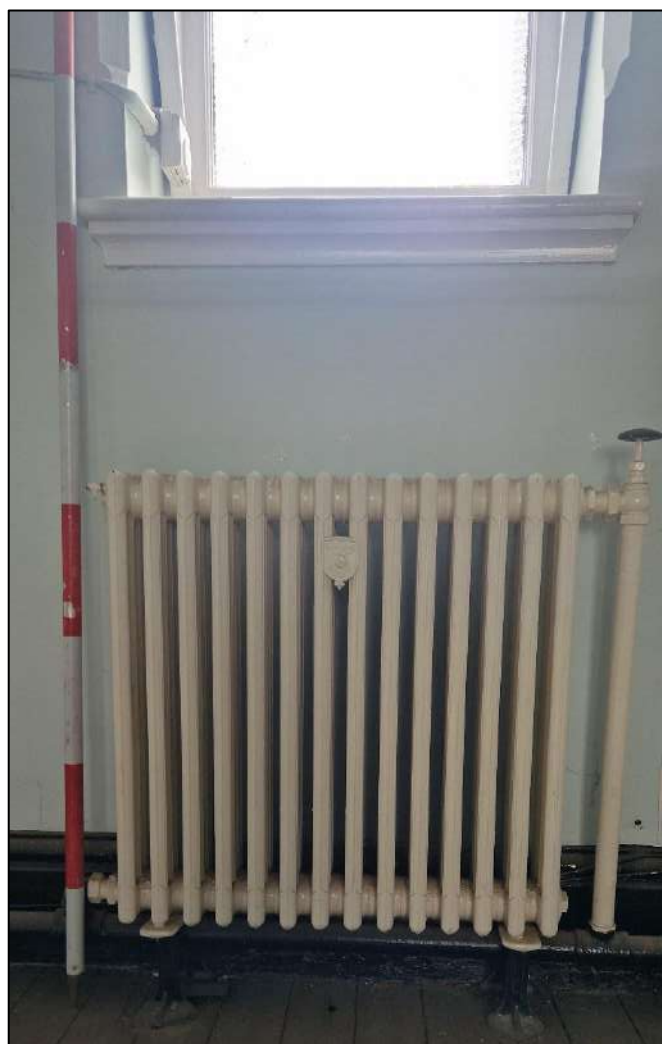
Plate 30. Radiator beneath window, view to the east, 2m scale.
