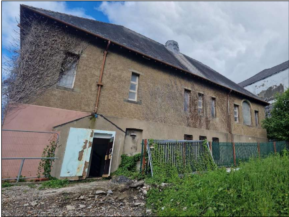
Plate 9. Rear elevation, view to the west-north-west
