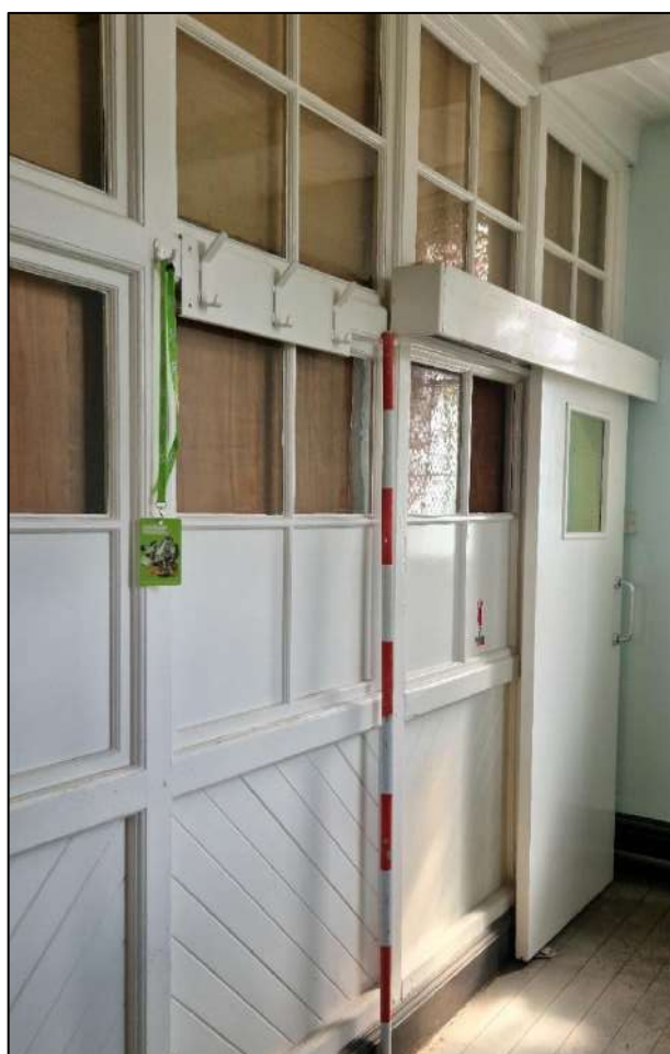
Plate 41. Sliding door on the north wall of the Project Room, view to the north-east, 2m scale.
