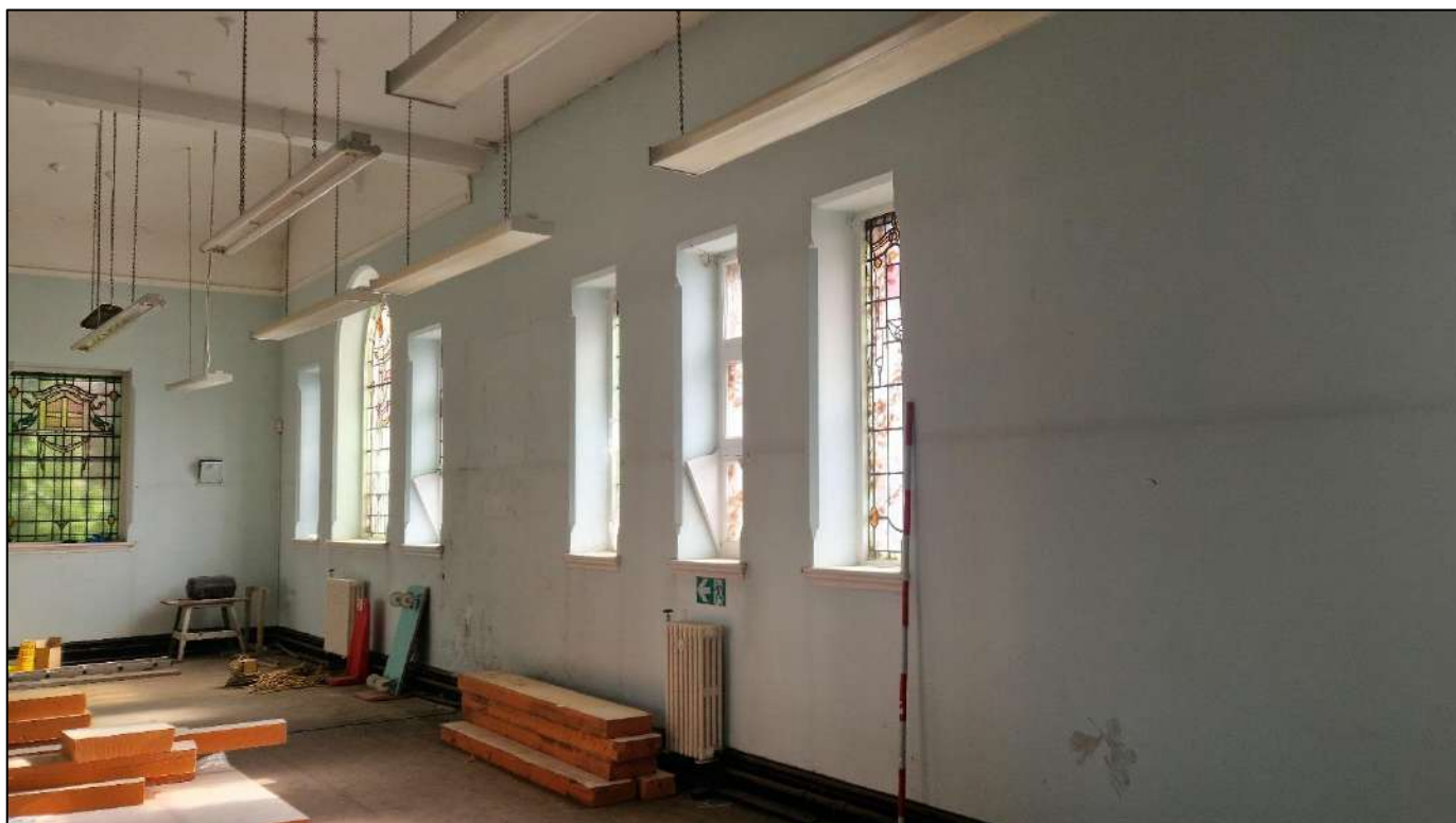
Plate 23. Central area, view to the north-east, 2m scale.
