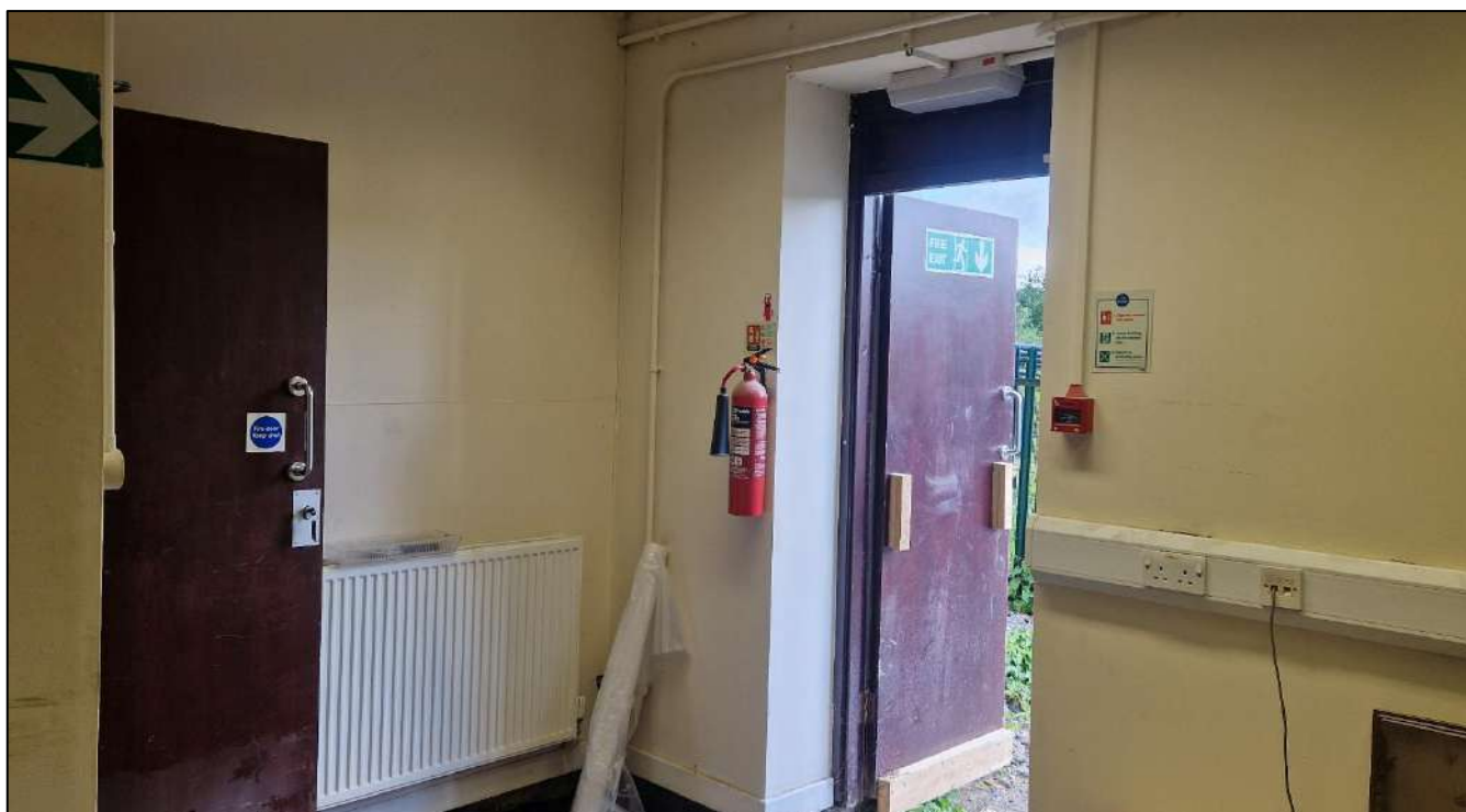
Plate 48. Rear doorway into the training Room, view to the north-east
