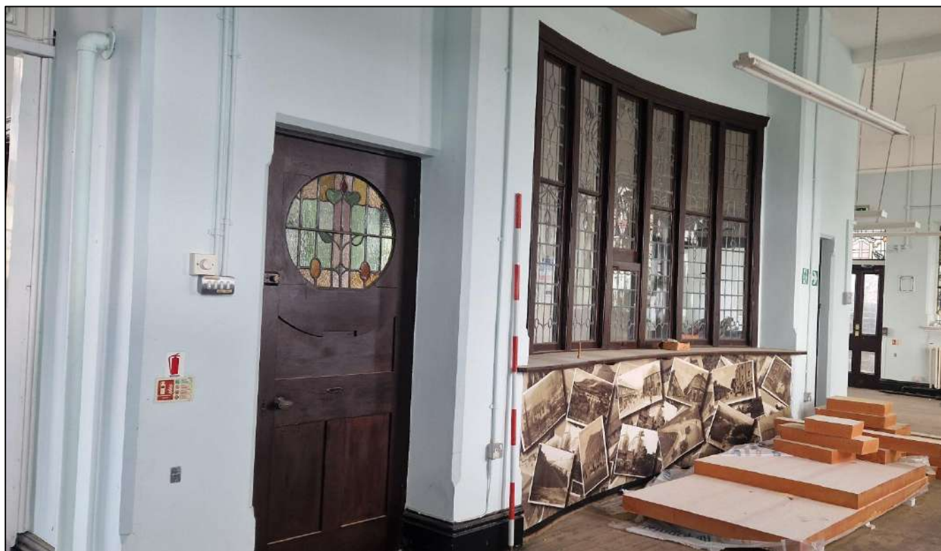
Plate 25. Rear of curved bay, view to the north-west, 2m scale.
