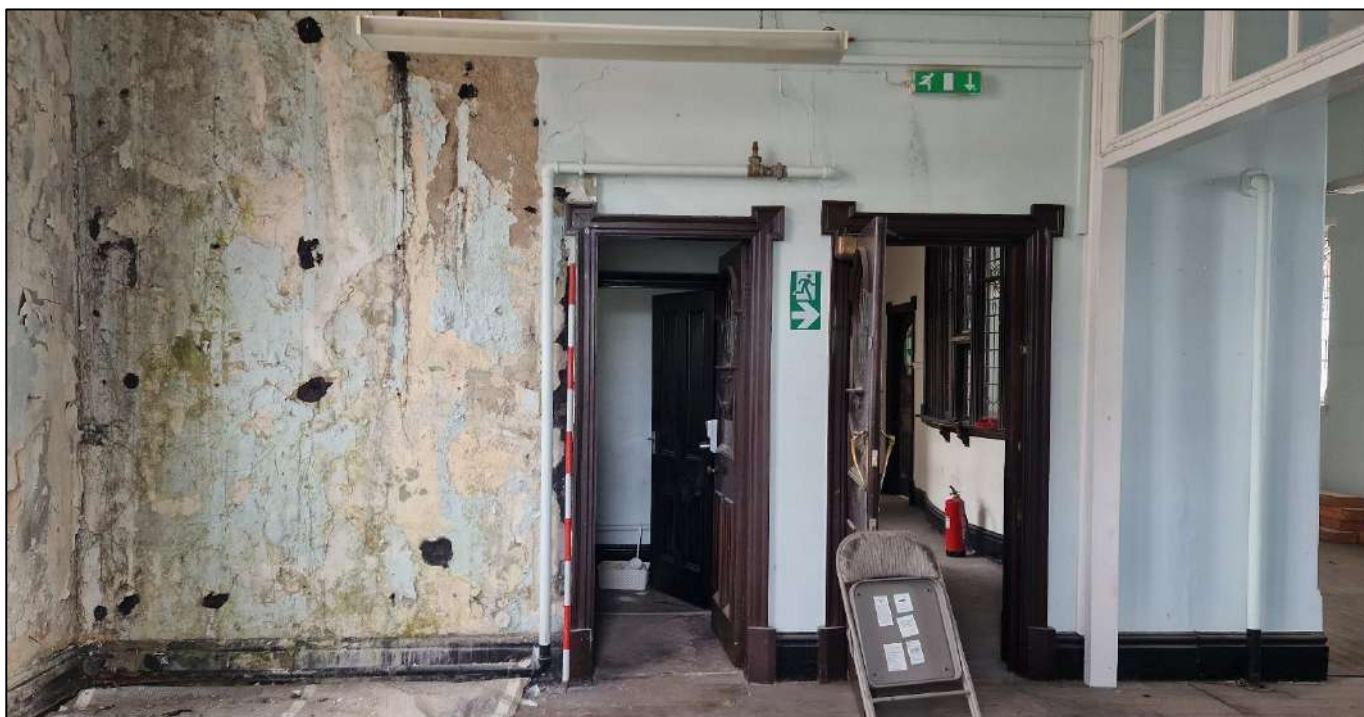
Plate 34. Doorway to the toilets and reception in the Junior Library, view to the north, 2m scale.
