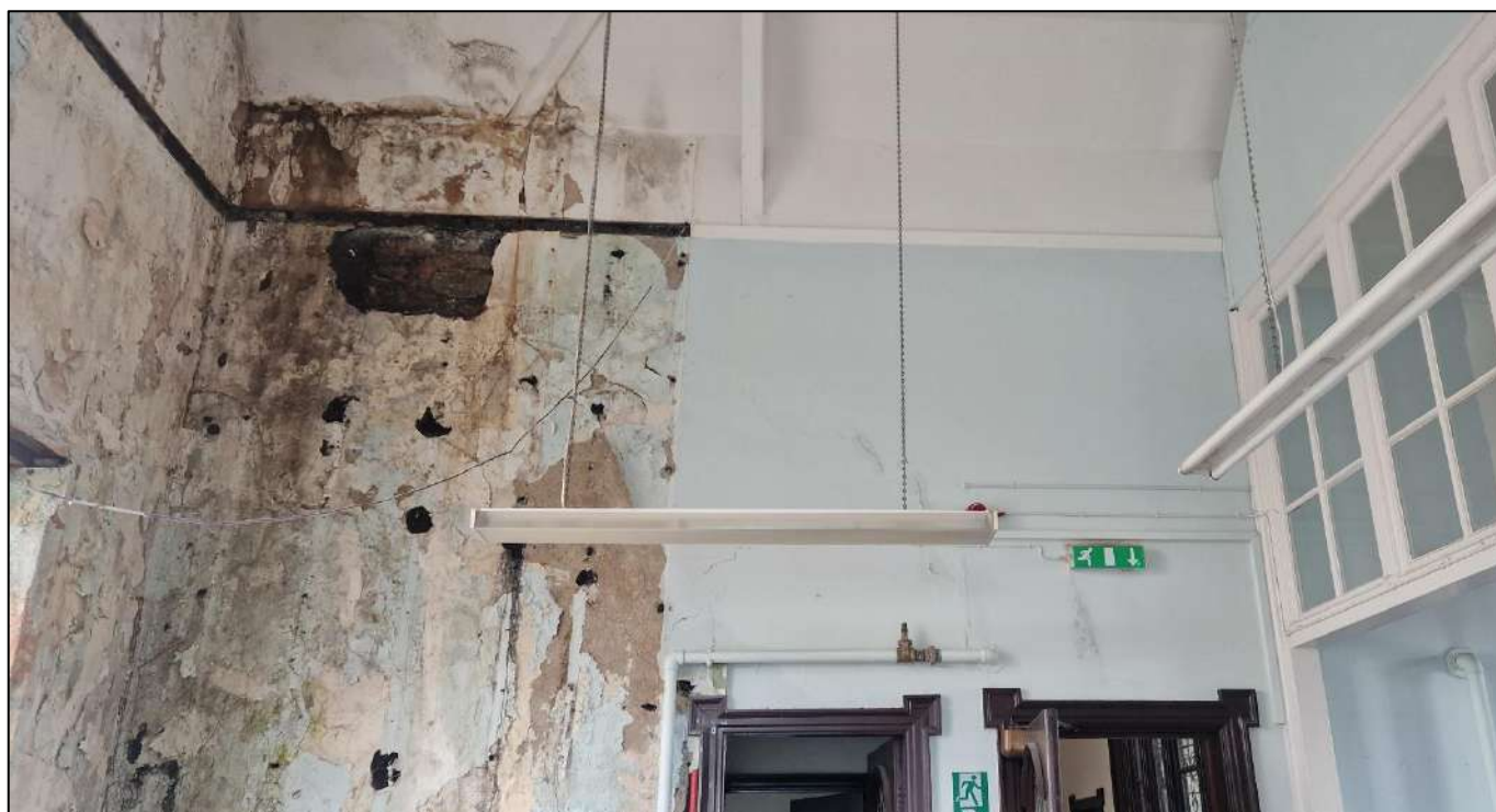
Plate 26. Southern section of the Library ceiling, view to the west, 2m scale.
