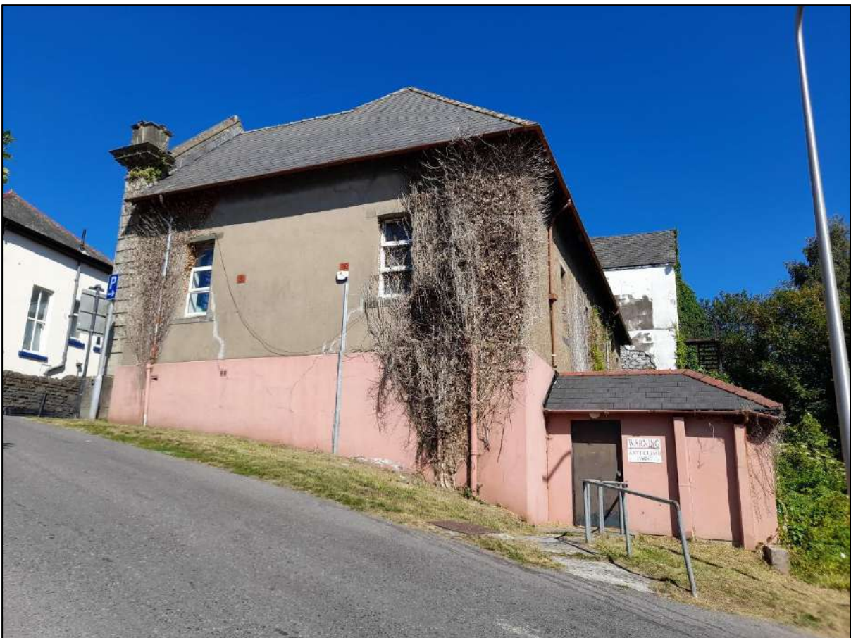
Plate 2. View, to the North of former extension, image taken for the HIA (AW, 2022)
