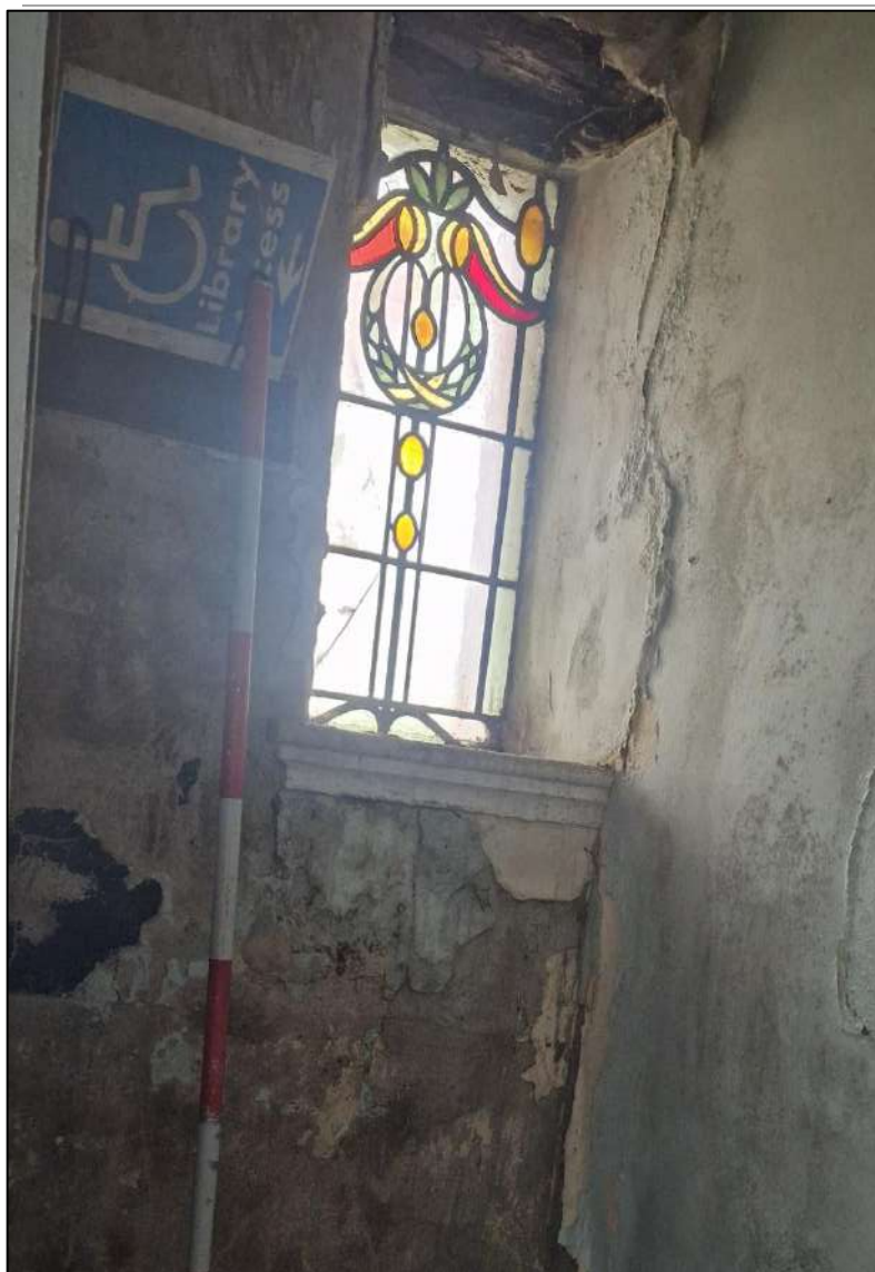
Plate 38. Window within small Cloakroom, view to the west, 2m scale.
