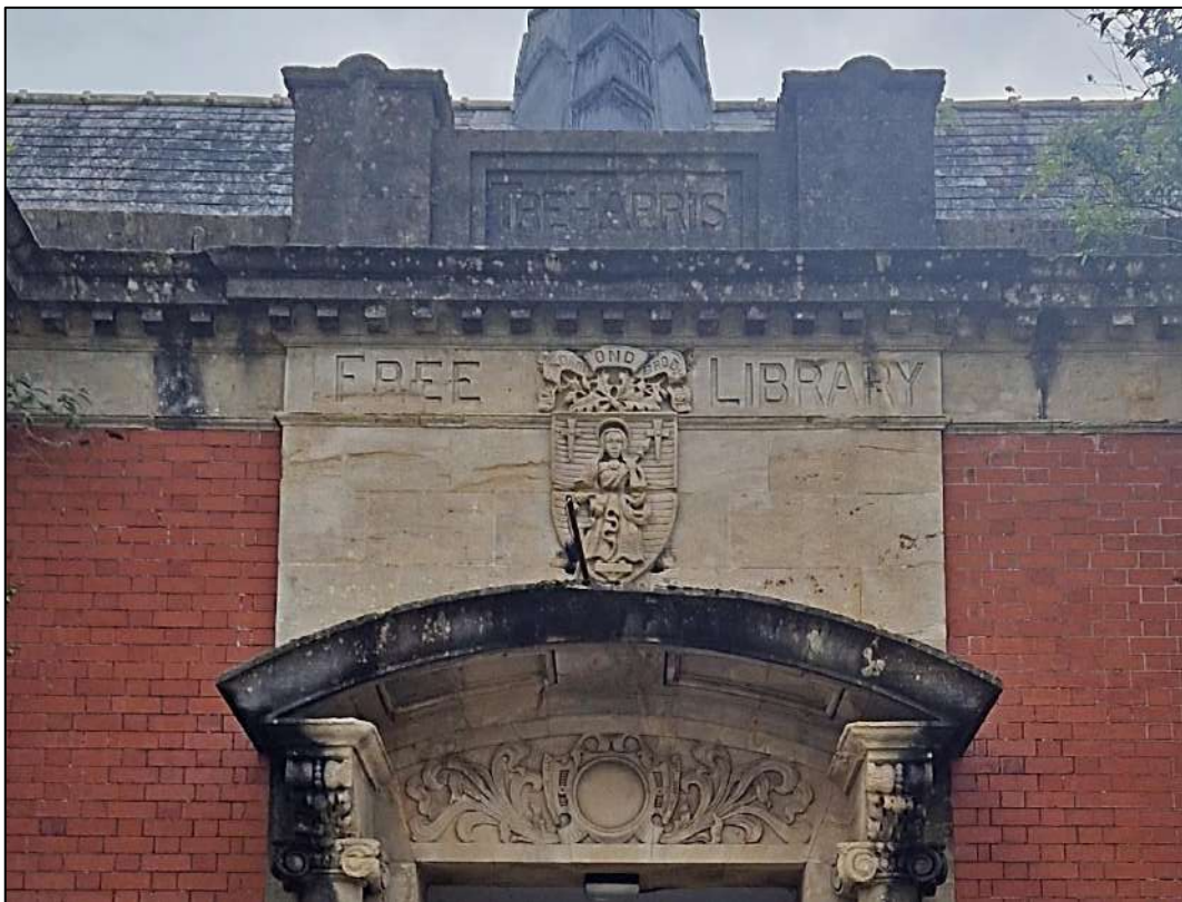
Plate 4. Entrance detail, view to the west
