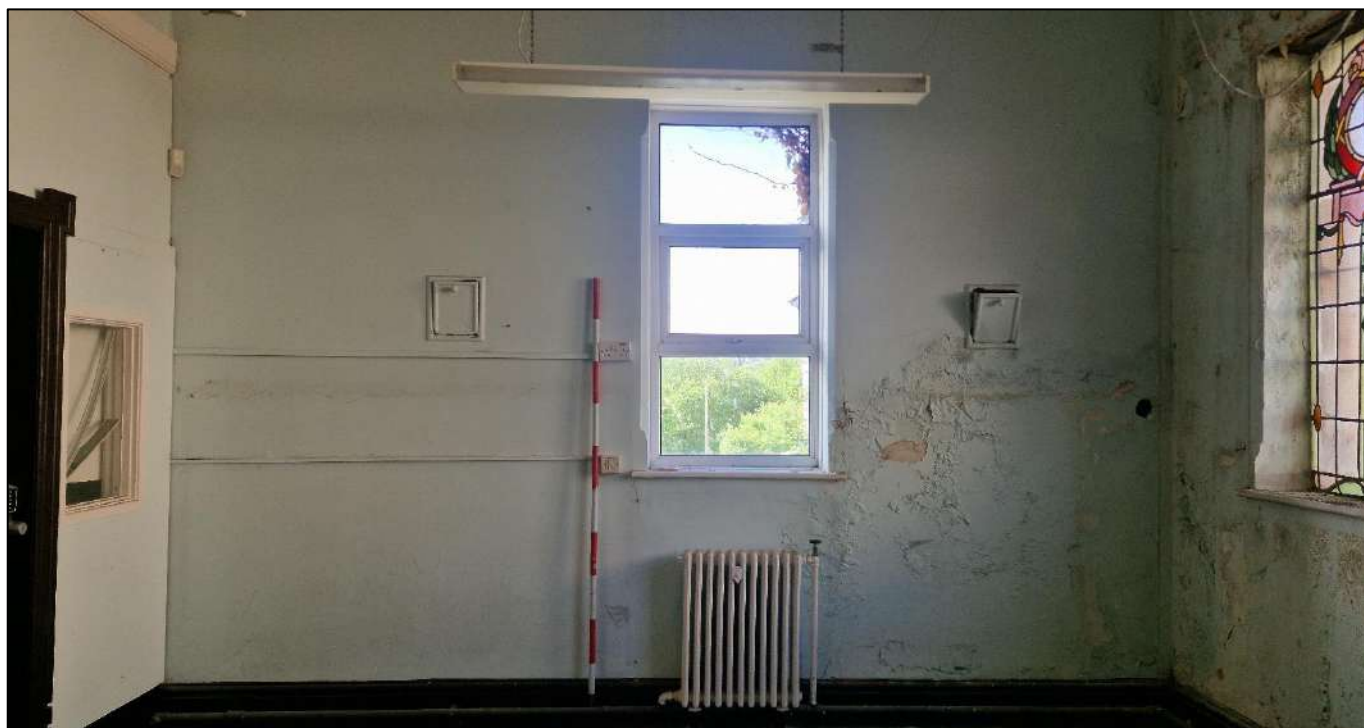
Plate 33. uPVC window on the southern wall of the Junior Library, view to the south, 2m scale.
