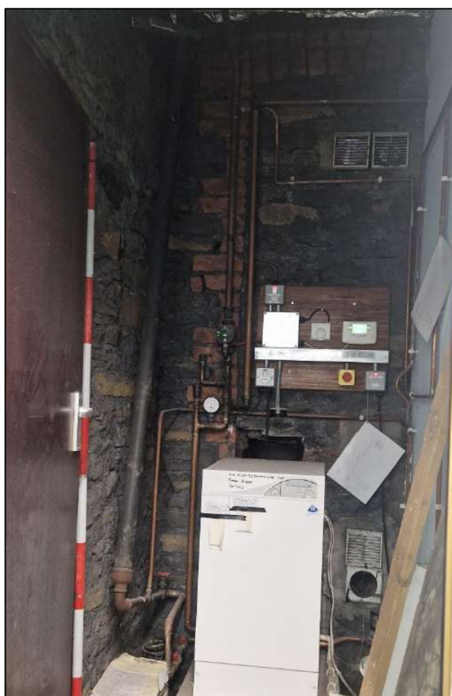
Plate 49. Boiler Room, view to the east, 2m scale.
