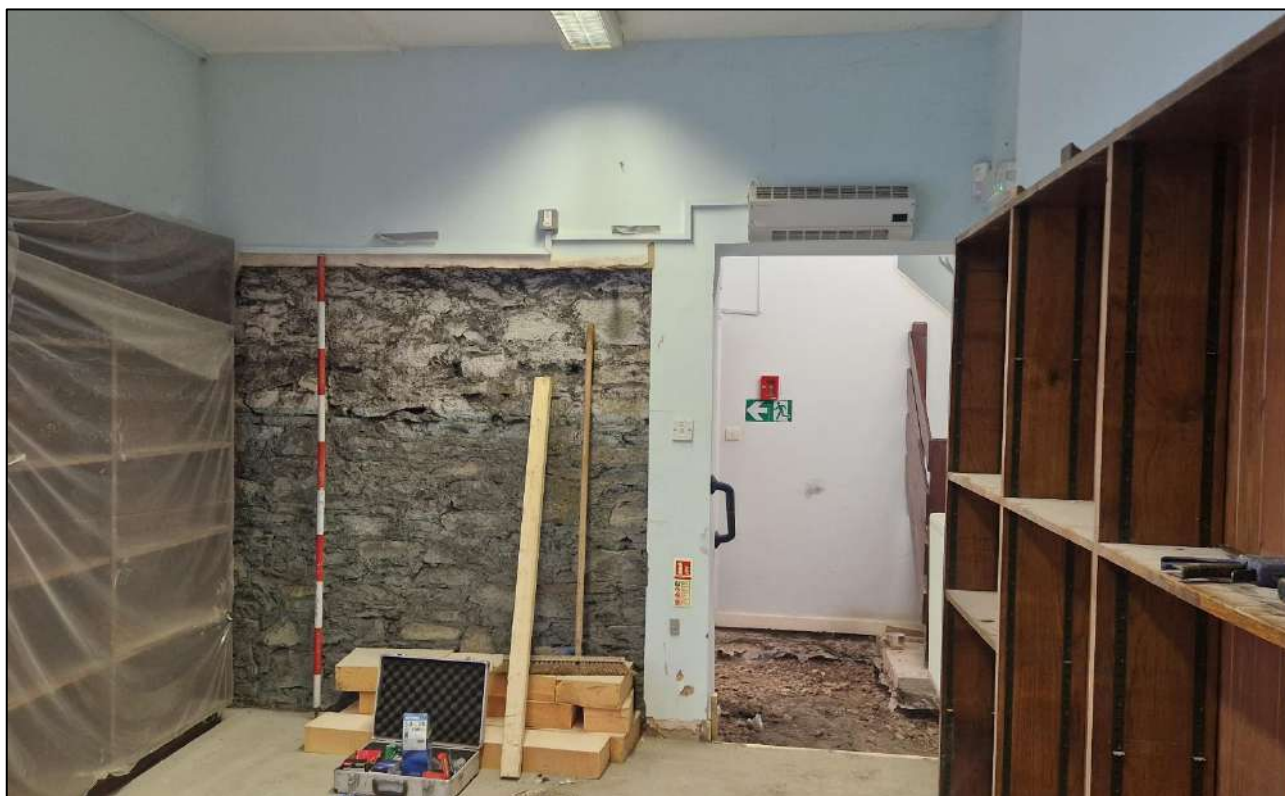
Plate 50. Opening between the Open Learning Room and the Basement Lobby, view to the south, 2m scale.
