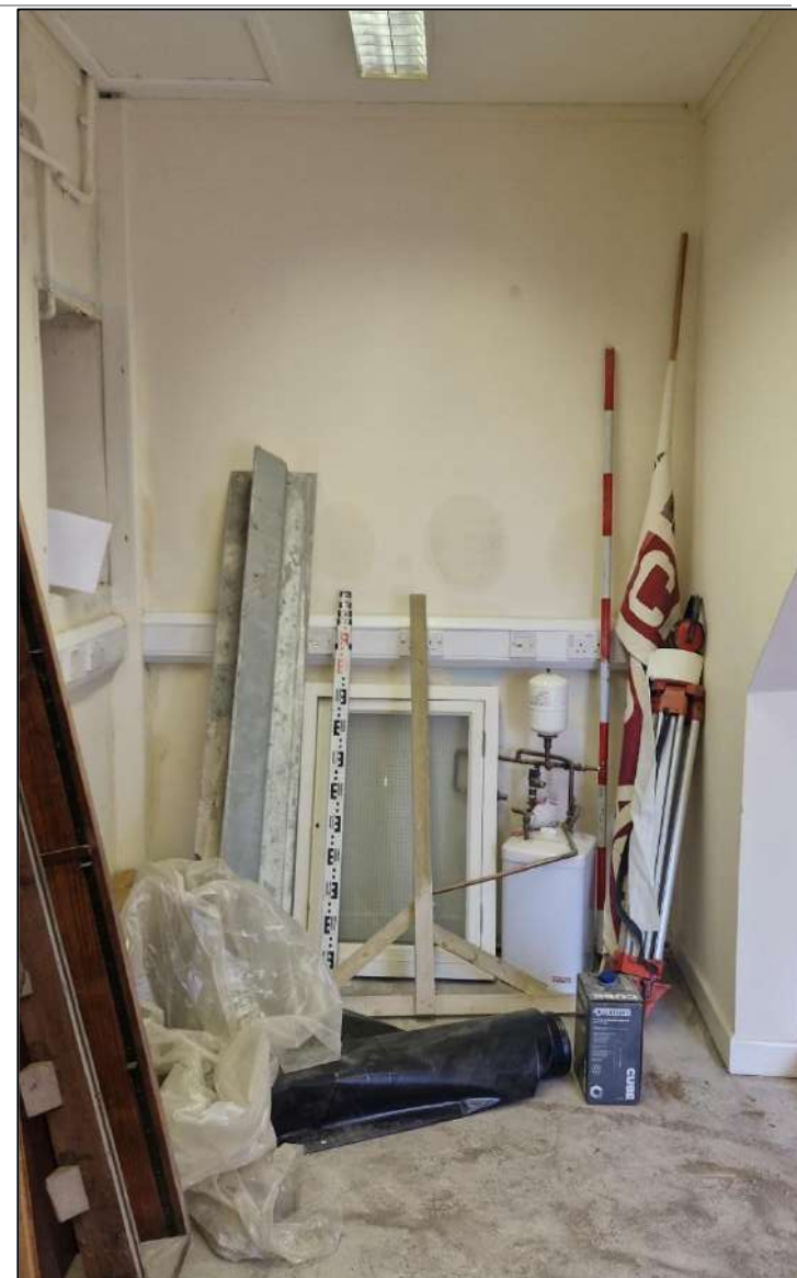
Plate 47. Training Room, view to the west, 2m scale.
