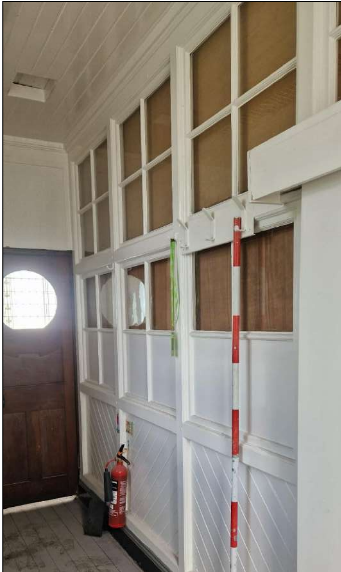
Plate 42. Panelled wall of the Project Room, view to the north-west, 2m scale.
