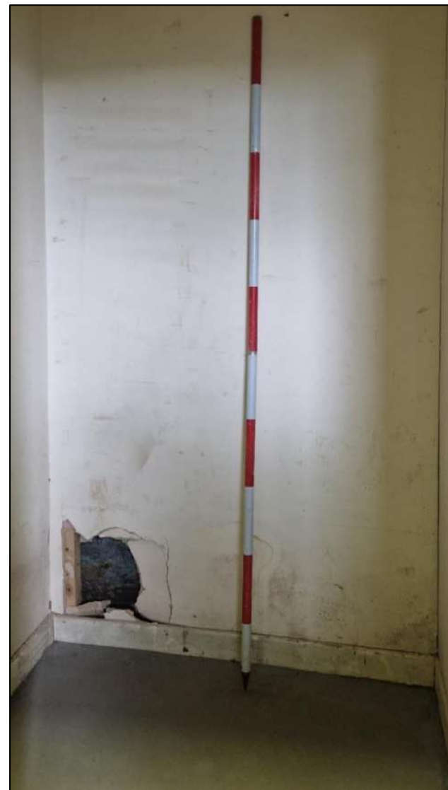
Plate 53. Cupboard in the Open Learning Room, view to the west, 2m scale.
