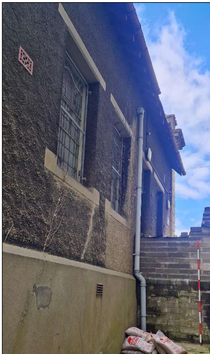
Plate 11. North elevation, view to the west, 2m scale.
