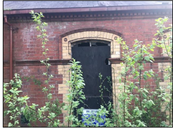
Photo 22 Open window on eastern elevation
