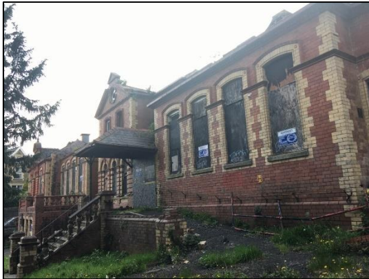
Photo 9 Front (south-eastern) elevation
