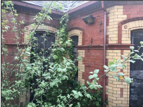
Photo 23 Open window on eastern elevation
