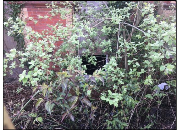
Photo 24 Open window on eastern elevation
