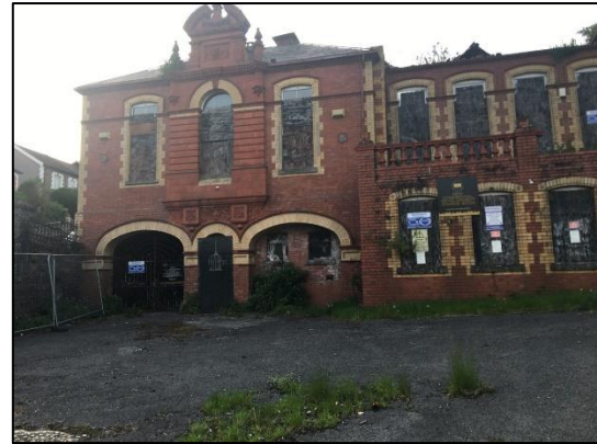
Photo 10 Front (southern) elevation
