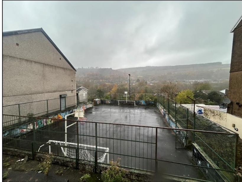
Photo 1 – view of court from Wesley Place
