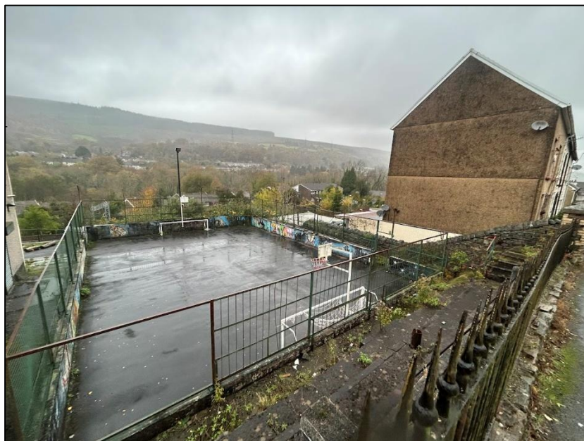
Photo 2 – view of former Church and side elevation of neighbouring house at No. 1 Wesley Place
