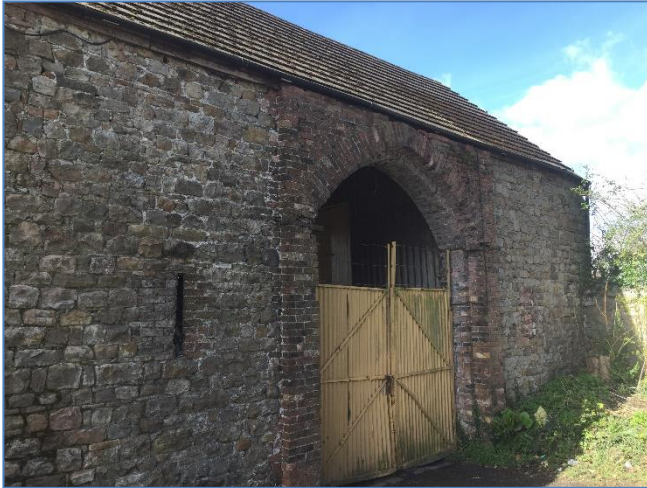
Photograph 1. Building B. The gated access on the northern elevation.
