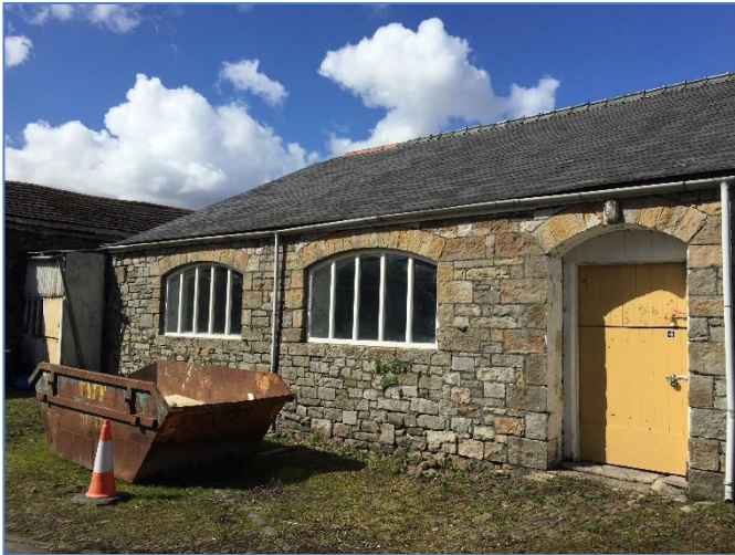
Photograph 13. Building C, southern half of the eastern elevation.
