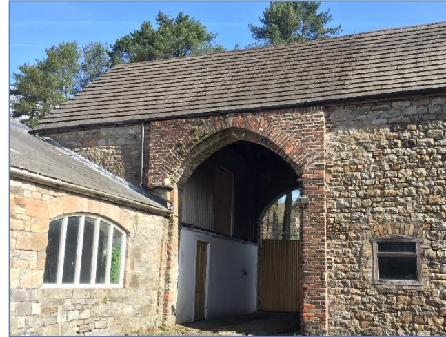
Photograph 2. Building B. The gated access on the southern elevation.
