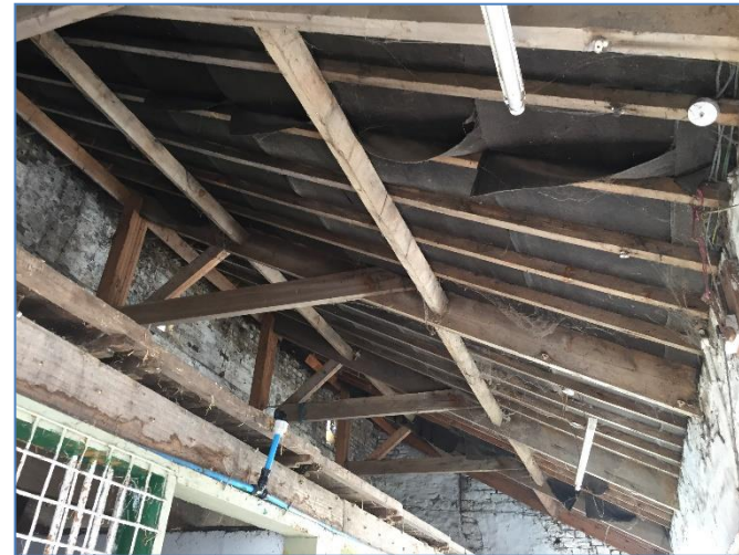
Photograph 16. Barn C. The internal roof construction and mezzanine loft.
