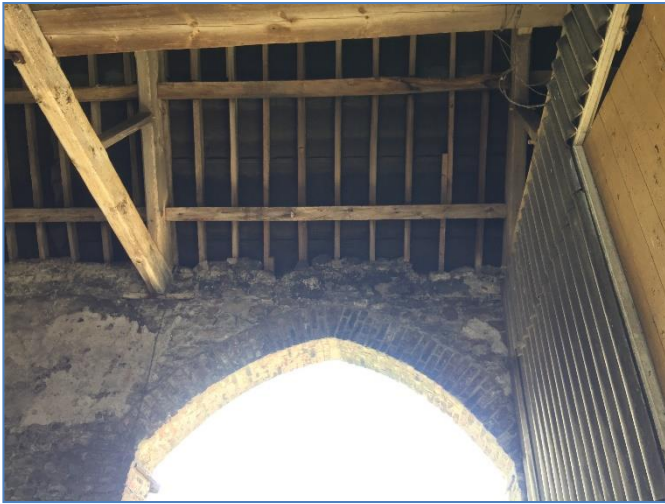
Photograph 5. Building B. The roof structure above the central gated section.
