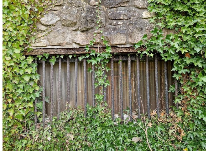
Ground floor window lintel
