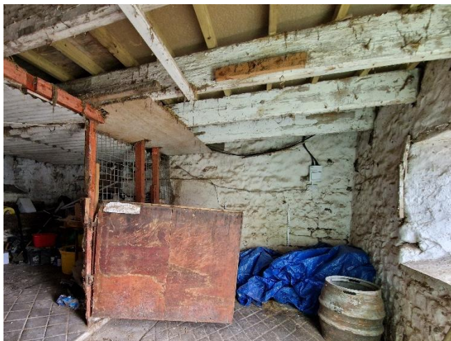
Bays D, E & F new joists over original beams
