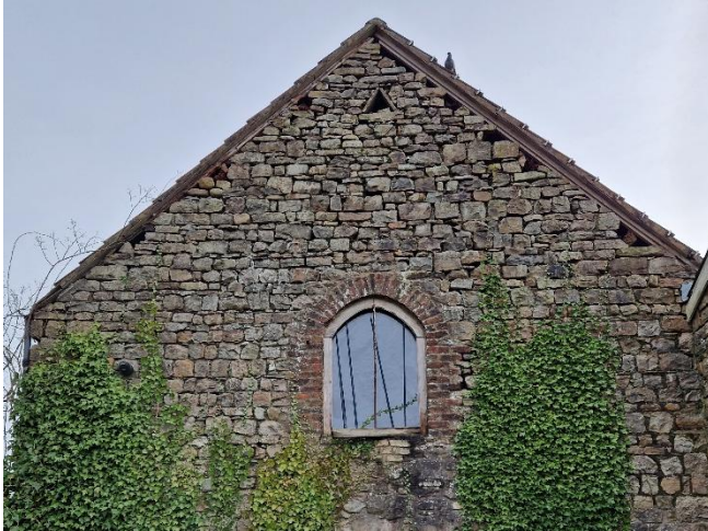
West gable high level masonry
