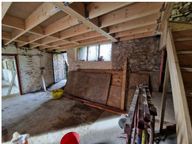
Bay A & C, complete replacement floor
