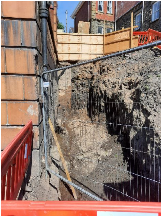
Above: Photographs indicating the extent of excavation required, with the Masonic Lodge visible in the background, to provide a safe environment for the construction of the replacement retaining wall.
