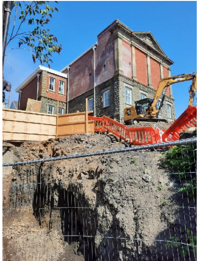
Above: Photographs indicating the extent of excavation required, with the Masonic Lodge visible in the background, to provide a safe environment for the construction of the replacement retaining wall.
