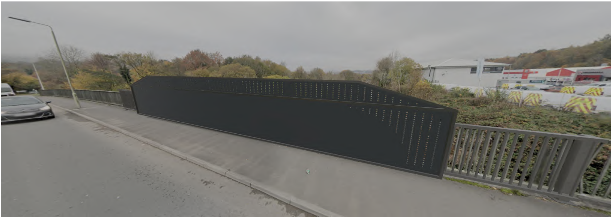
ELEVATION ON SOUTHERN PARAPET
