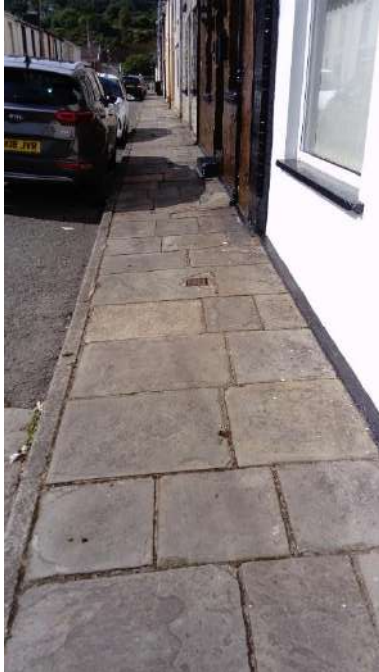
Plate 3.6: Footways along Cardiff Street
