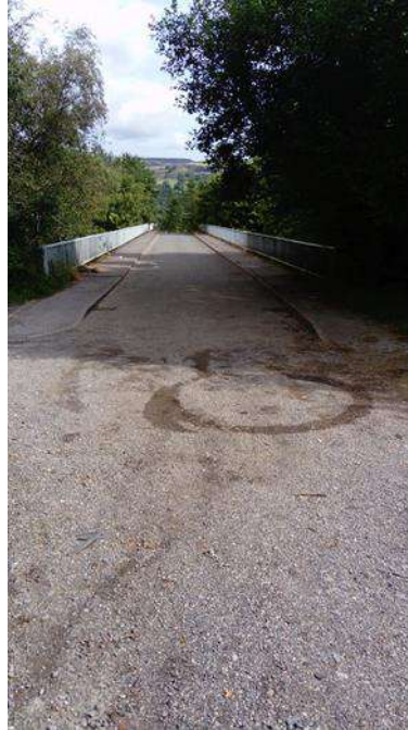
Plate 3.2: Bridge over A470
