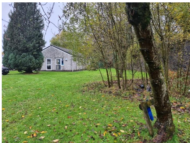
Figure 9 – Looking west towards existing small building at the west of the site.
