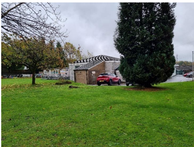
Figure 7 – Looking south towards existing school building.
