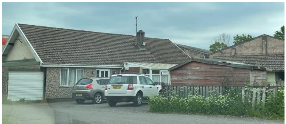
Photograph of Riverside Bungalow
