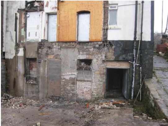
Plate 7: Rear of La Bodega, showing open area following removal of extension and lean-to structures
