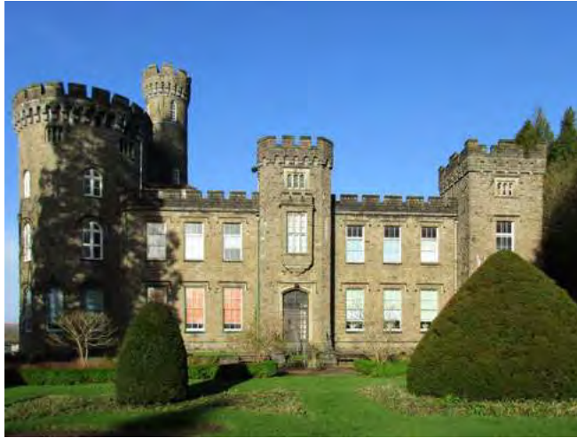
East elevation and former family entrance
