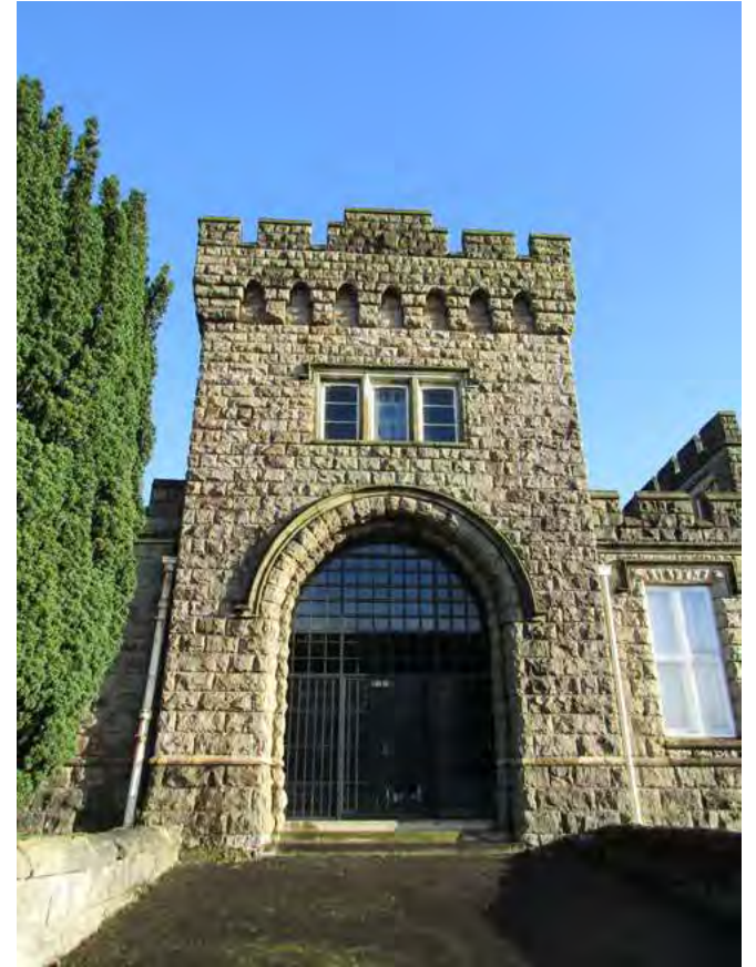
West gatehouse (former Stable entrance)
